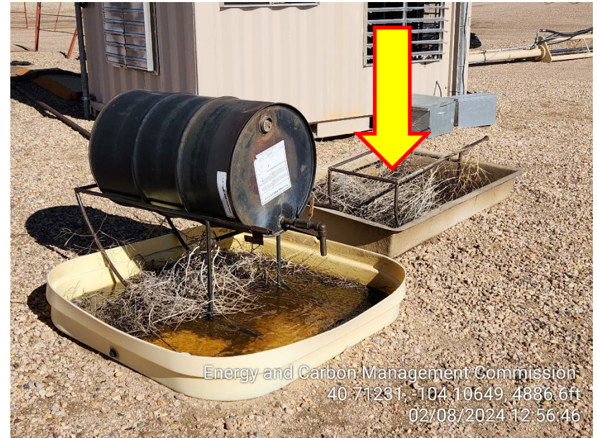
Photo 14 – Unused Secondary Containment at 32-68HN Wellsite
