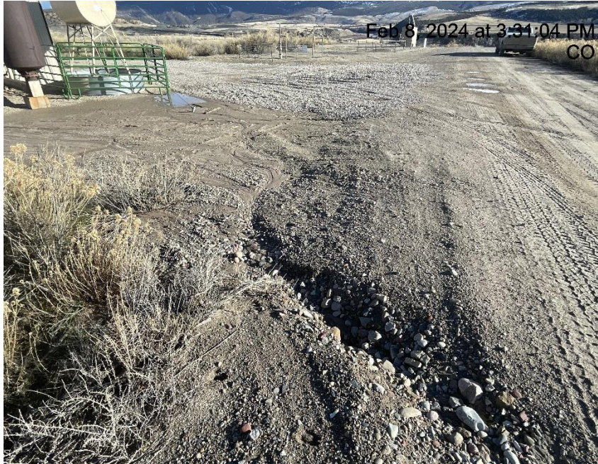
Photo # 5605 Erosion & transport of sediment onto location/insufficient BMP's/insufficient run on/runoff controls
