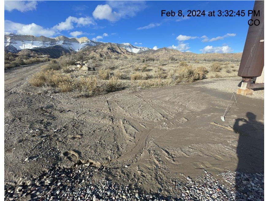
Photo # 5612 Erosion & transport of sediment onto location/insufficient BMP's/insufficient run on/runoff controls
