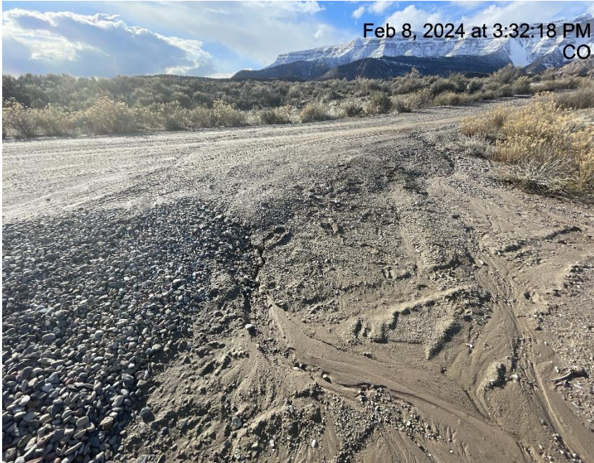
Photo # 5609 Erosion & transport of sediment onto location/insufficient BMP's/insufficient run on/runoff controls
