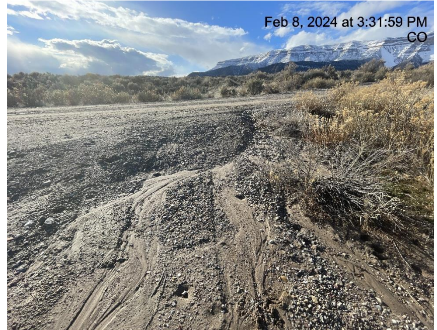
Photo # 5608 Erosion & transport of sediment onto location/insufficient BMP's/insufficient run on/runoff controls
