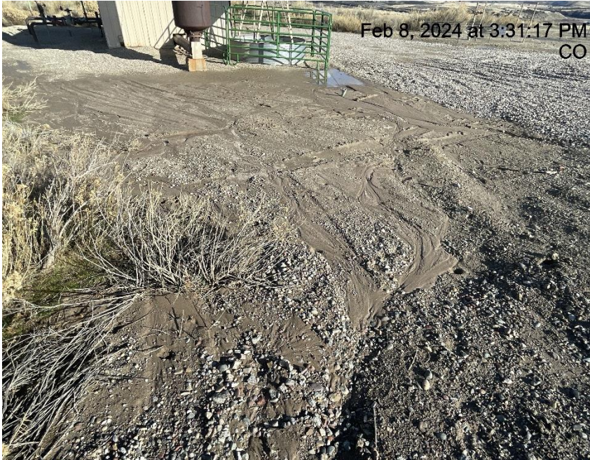
Photo # 5607 Erosion & transport of sediment onto location/insufficient BMP's/insufficient run on/runoff controls
