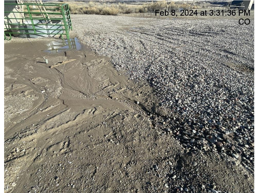
Photo # 5610 Erosion & transport of sediment onto location/insufficient BMP's/insufficient run on/runoff controls
