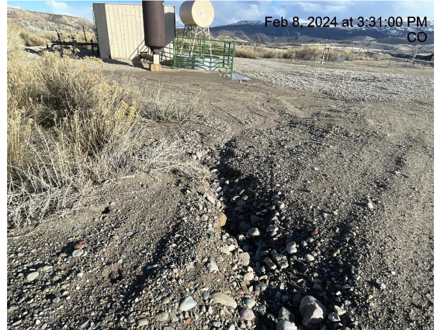
Photo # 5606 Erosion & transport of sediment onto location/insufficient BMP's/insufficient run on/runoff controls
