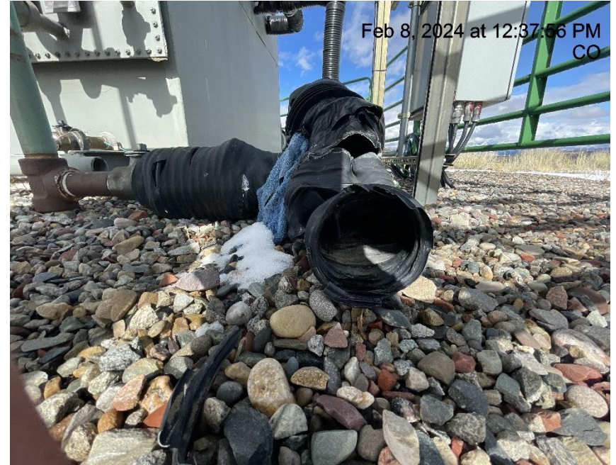
Photo # 6107 Flowline heating insulation open ended/wildlife hazard/available for entry by wildlife
