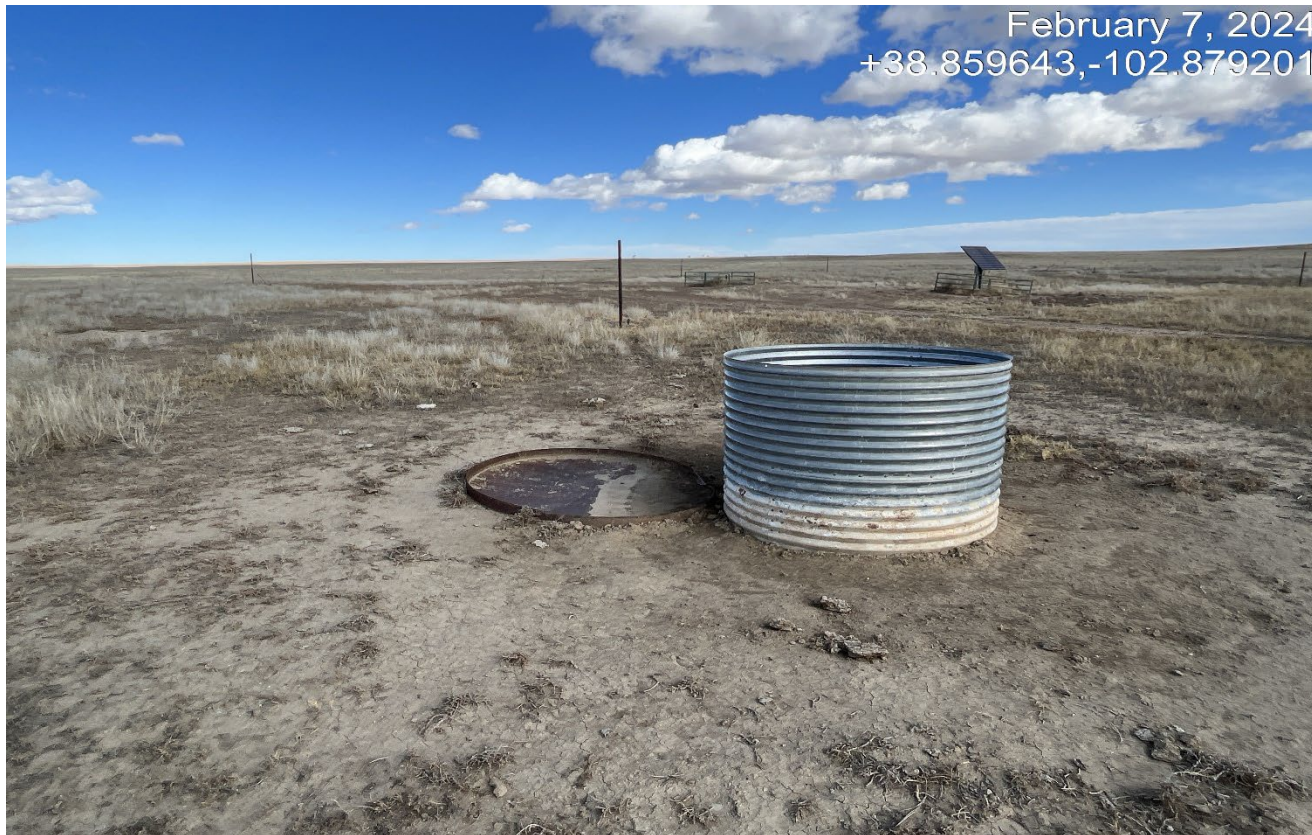
Photo 7. Southwest side of the location facing northeast. There is a pipeline cellar with the lid off laying on the ground.
