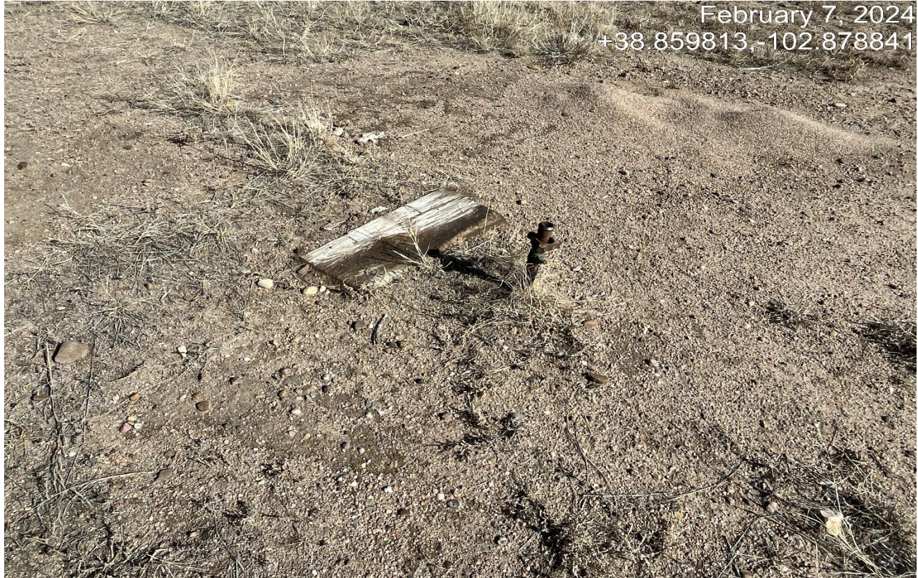
Photo 4. The pipe riser is not capped and is is unused which needs to be removed.
