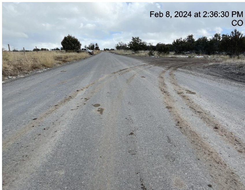
Photo # 6188 Insufficient tracking BMP's/tracking off lease road & onto CR 336 (Jenkins Cutoff)
