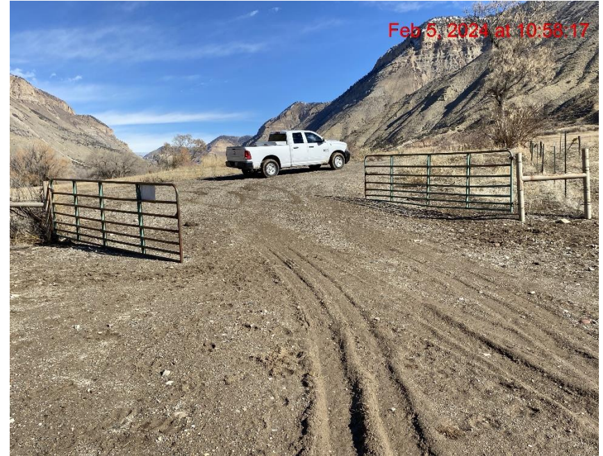
Insufficient Vehicle Tracking BMPs at Location Entrance/Exit – Photo #09143
