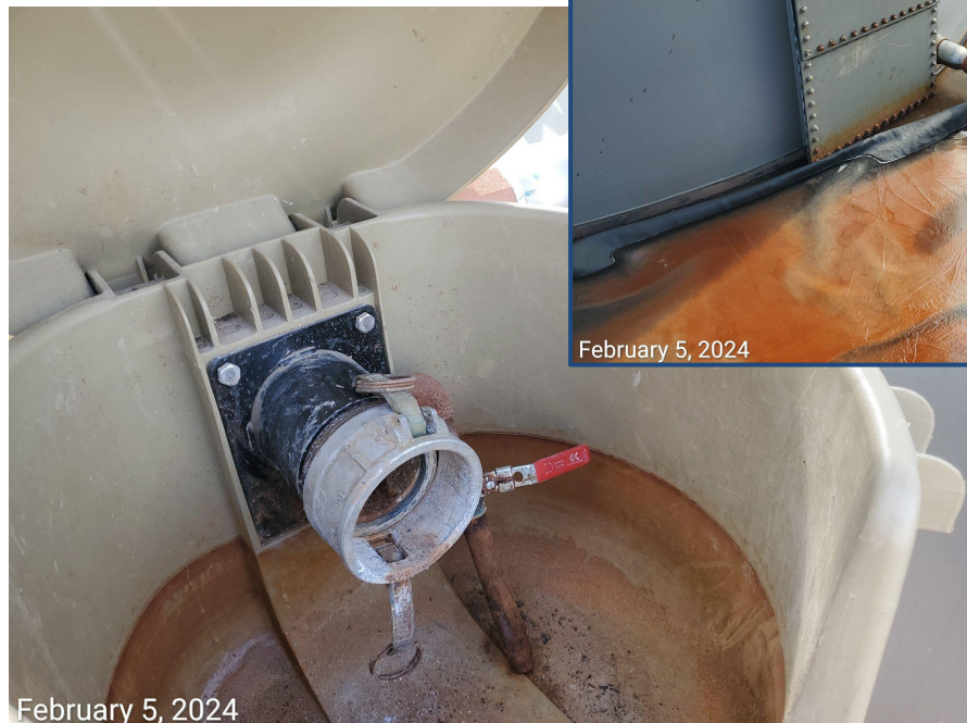
Photo 4: Lines at tanks lack cap/plug.
