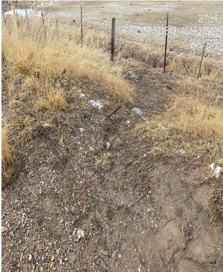
Photo 6. View of gully erosion forming in the western interim reclamation area, with old wattle stakes observed in the ground.
