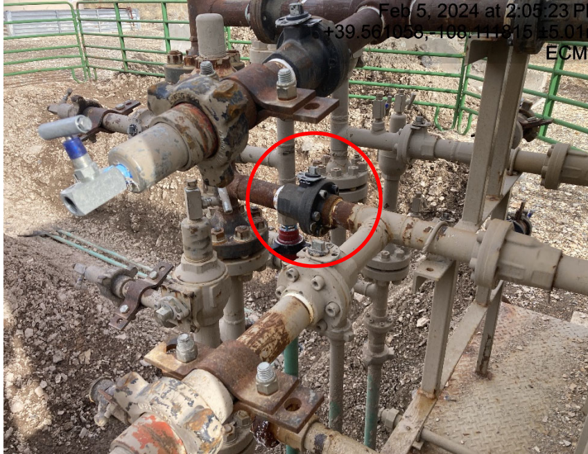
Valve leaking
