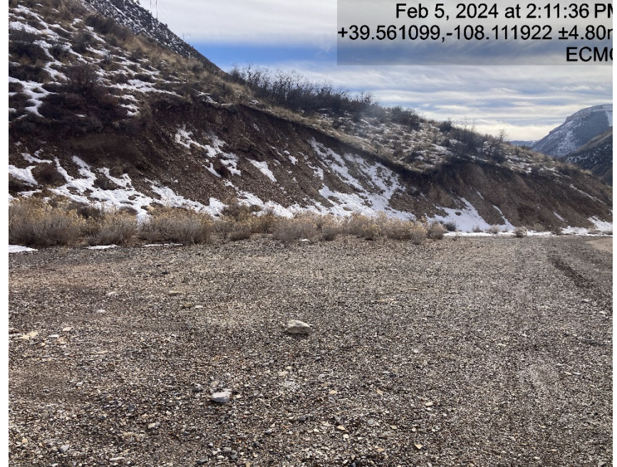
Cut slope is eroding
