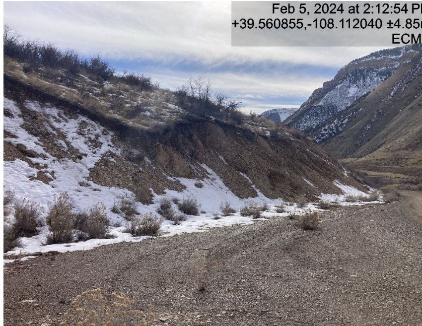
Cut slope is eroding
