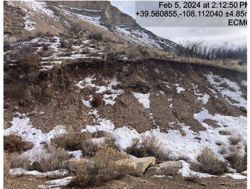
Cut slope is eroding
