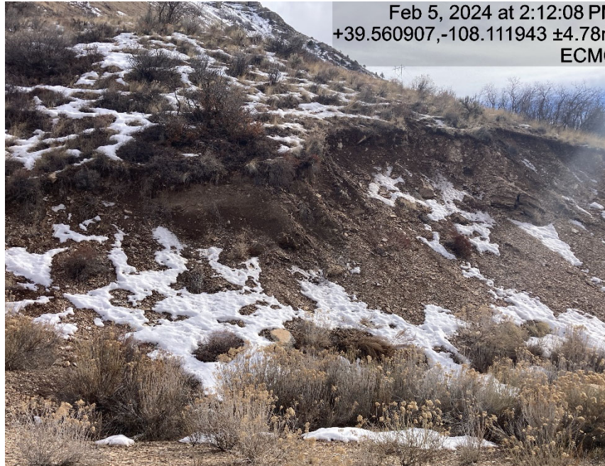
Cut slope is eroding
