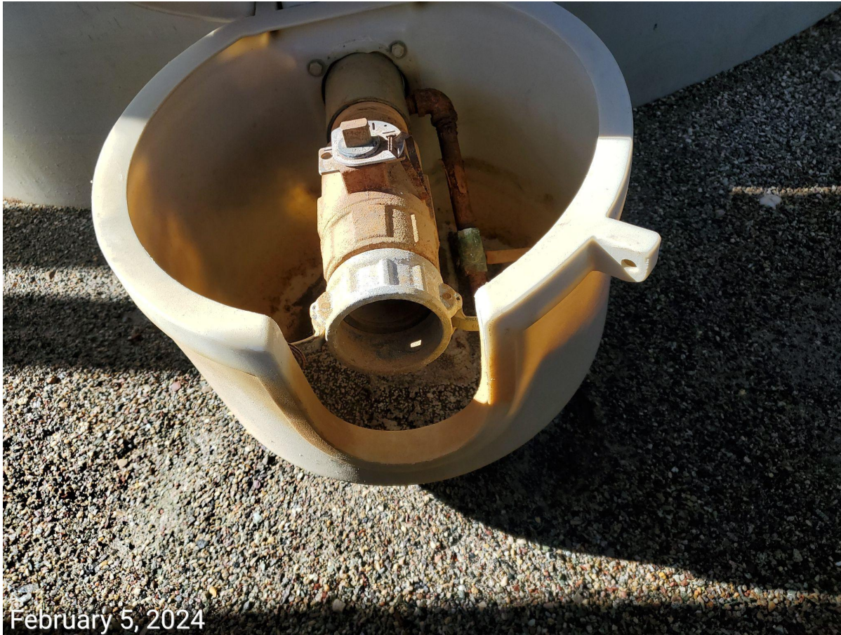
Photo 9: Lines at tanks lack cap/plug.
