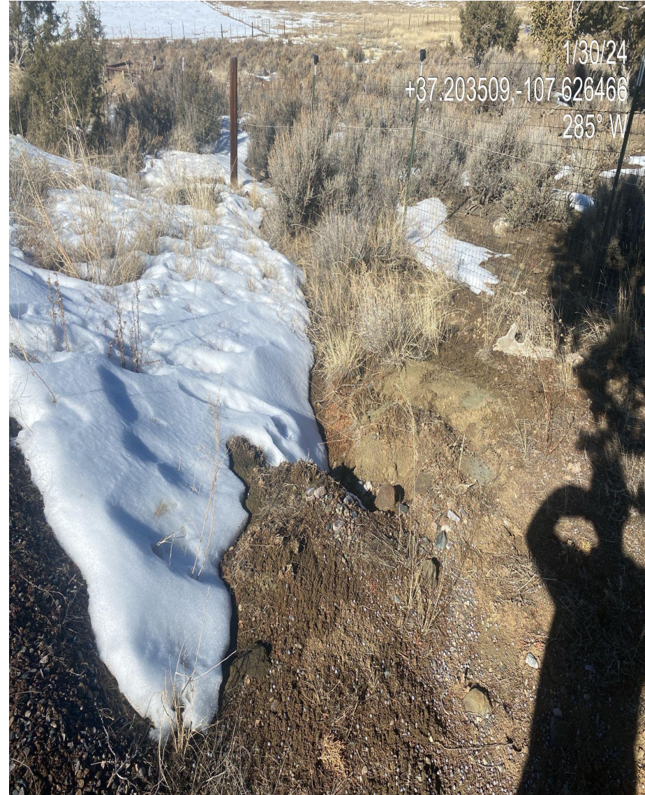
Photo 5. Rill erosion forming along the access road at the access point of the disturbance.
