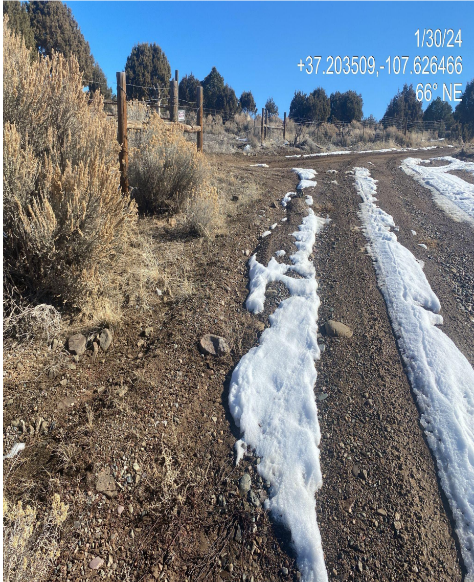
Photo 5. Rill erosion forming along the access road at the access point of the disturbance.
