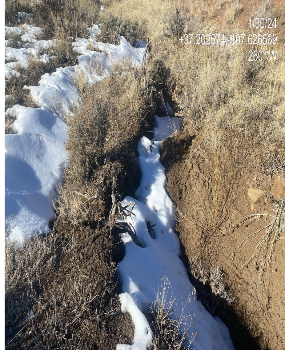
Photo 4. Gully erosion forming downhill of current stormwater BMPs in the southern interim reclamation area.
