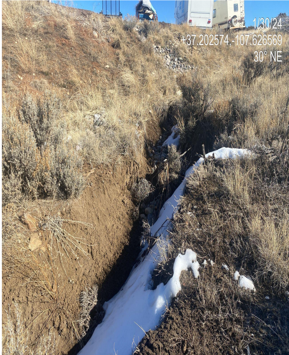
Photo 4. Gully erosion forming downhill of current stormwater BMPs in the southern interim reclamation area.
