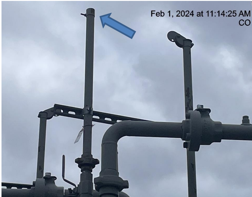
Photo # 4995 Rupture disc vent line lacks cap
