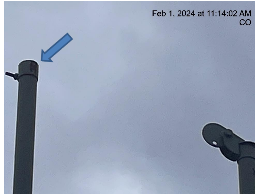
Photo # 4996 Rupture disc vent line lacks cap
