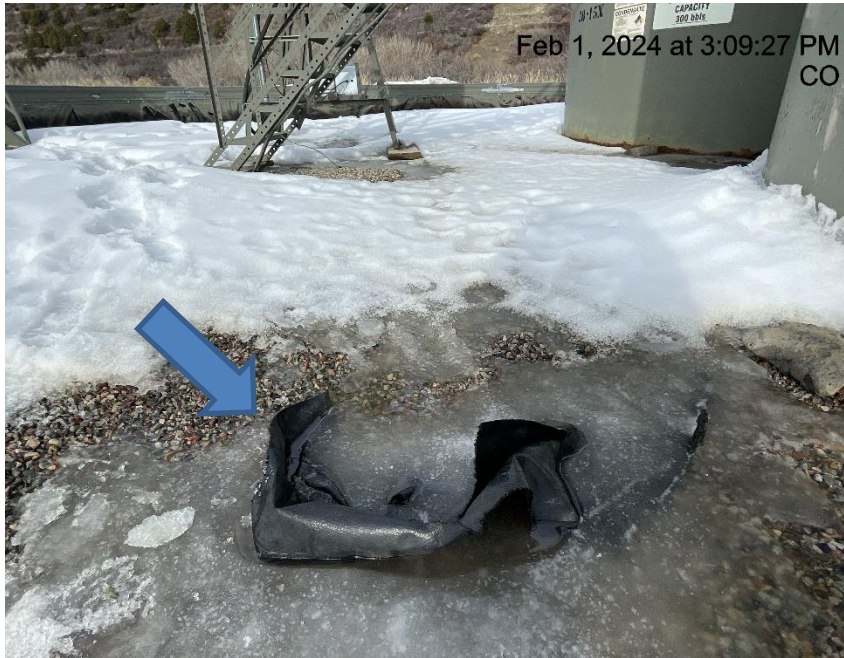
Photo # 5409 Possible tear in base of secondary containment liner
