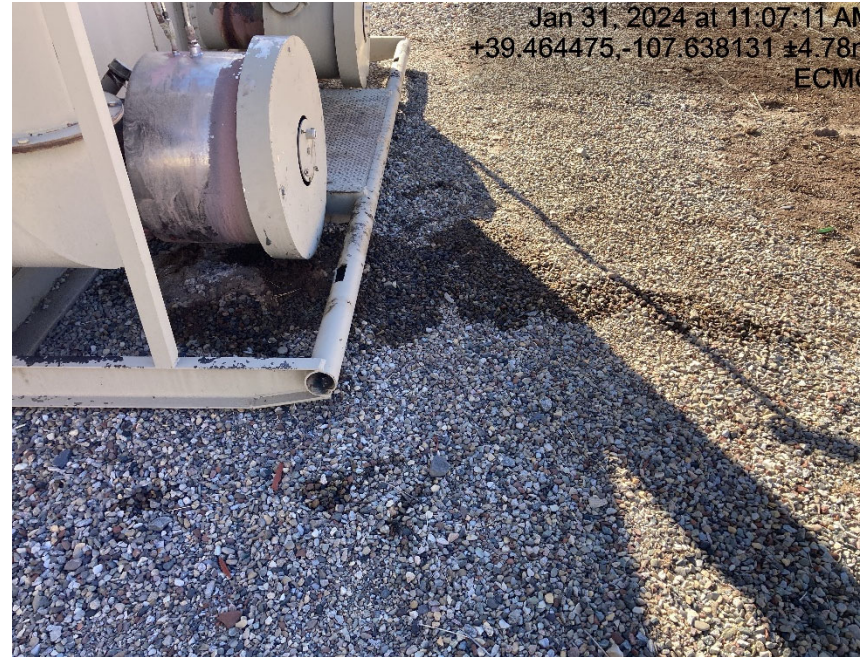
Staining behind separator
