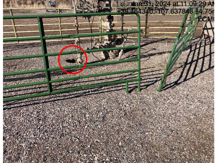
Open hole next to well head and fencing is open
