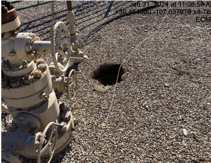
Open hole next to well head
