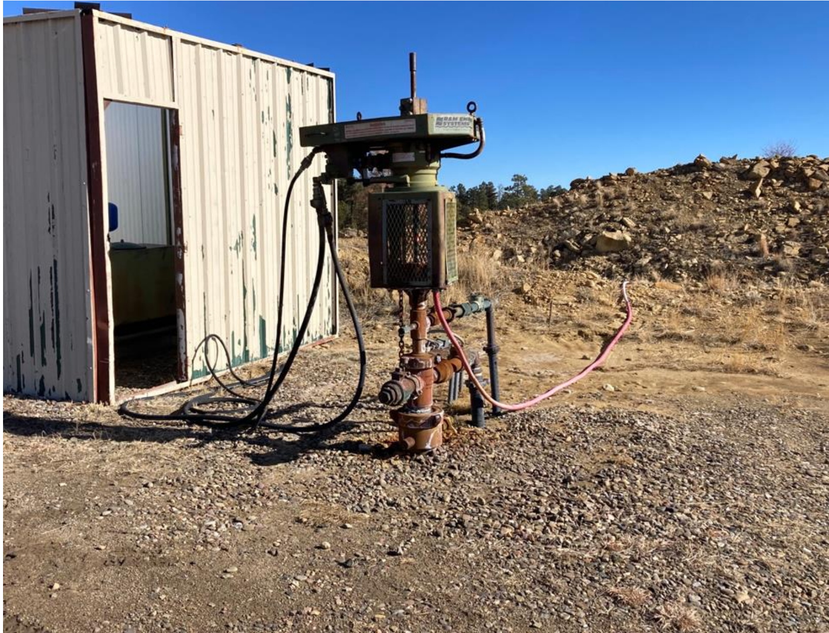
PHOTO 1: THE WELLHEAD PACKINGS WERE REPLACED AND THE STUFF BOX WAS SECURELY FASTENED TO STOP THE WATER LEAK. ANY IMPACTED SOIL HAS BEEN REMOVED FROM LOCATION. ALL EQUIPMENT HAS RECEIVED MAINTENACE TO ENSURE GOOD MECHANICAL OPERATING CONDITION.
