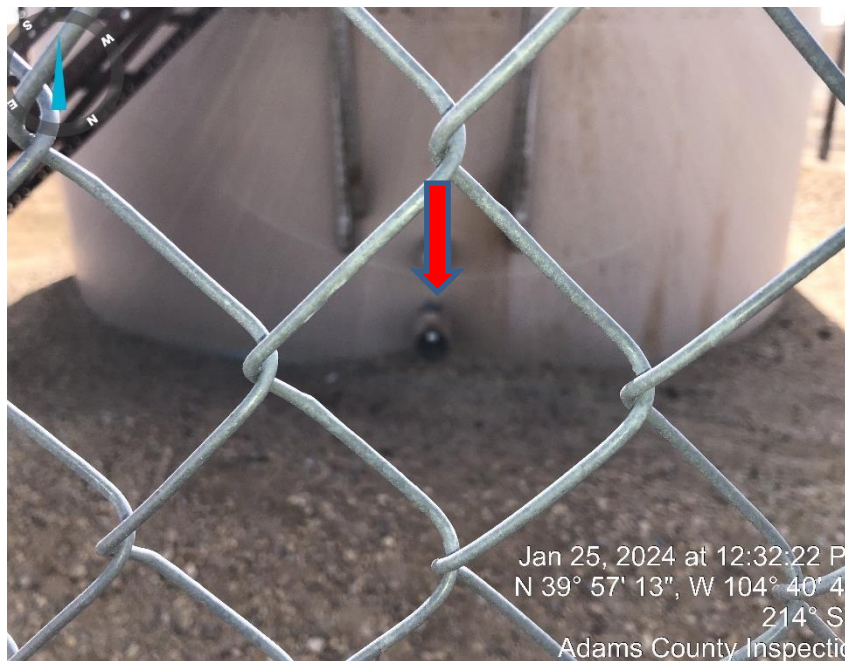
Photo #2 No bull plug in load out line.
