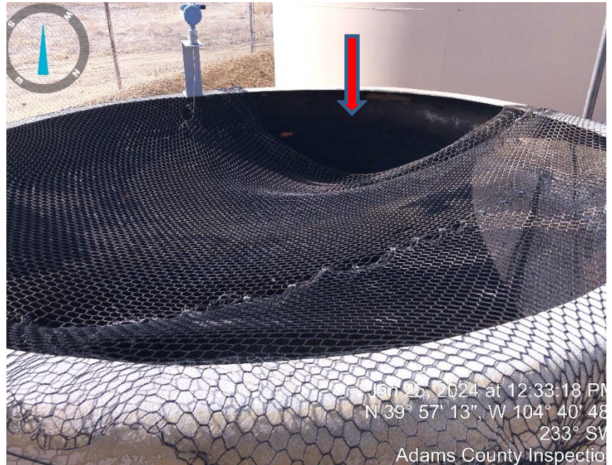
Photo #4 Net over open top P/W tank falling in tank.
