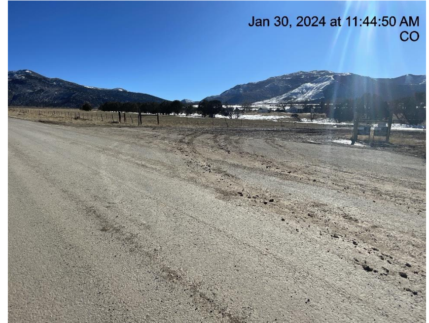
Photo # 4827 Insufficient tracking BMP's/tracking off location & onto to CR 306 (Spring Creek RD)
