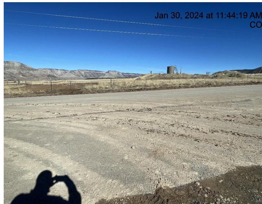
Photo # 4823 Insufficient tracking BMP's/tracking off location & onto to CR 306 (Spring Creek RD)
