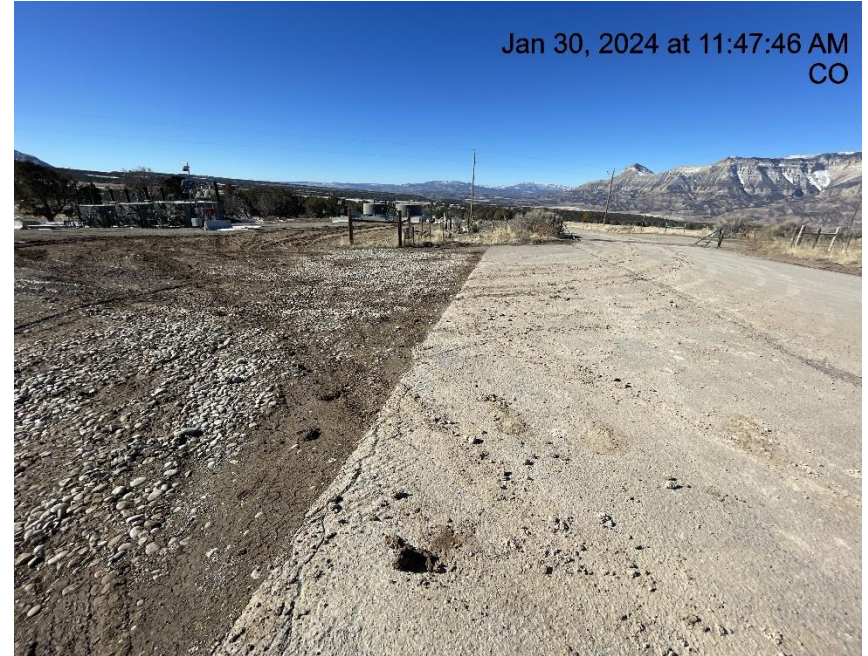
Photo # 4843 Insufficient tracking BMP's/tracking off location & onto to CR 306 (Spring Creek RD)
