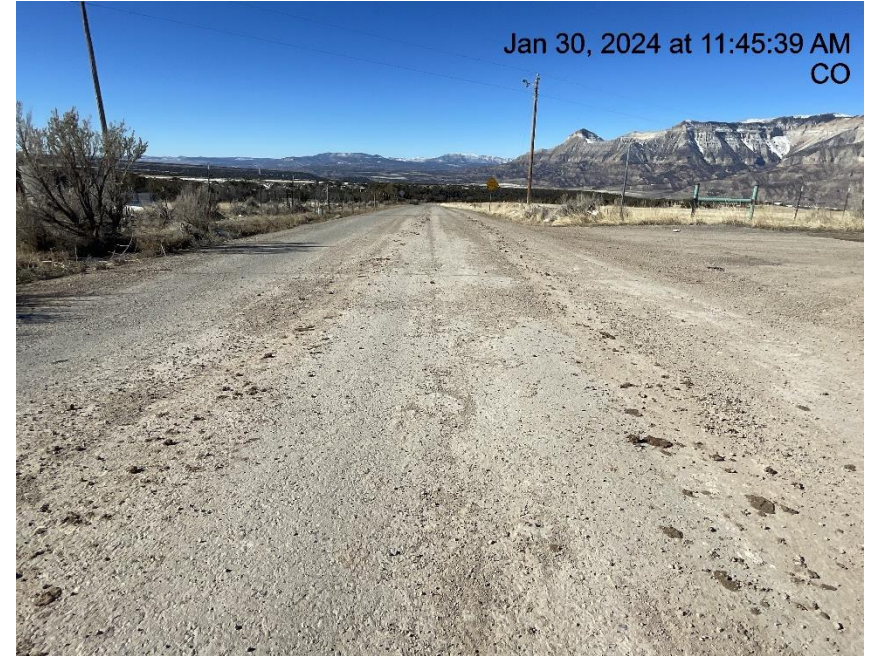
Photo # 4835 Insufficient tracking BMP's/tracking off location & onto to CR 306 (Spring Creek RD)
