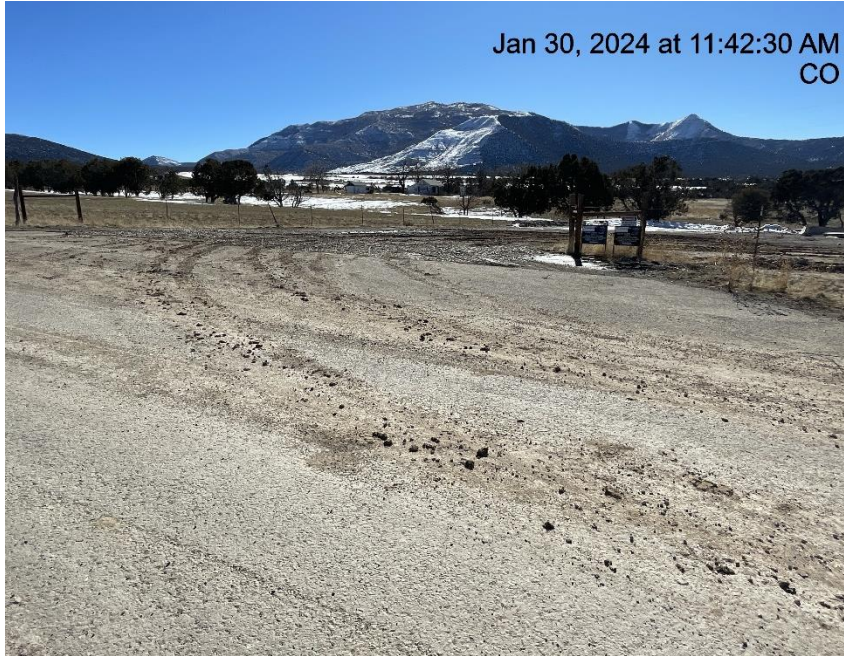
Photo # 4824 Insufficient tracking BMP's/tracking off location & onto to CR 306 (Spring Creek RD)
