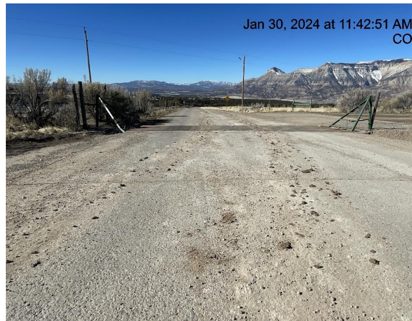
Photo # 4831 Insufficient tracking BMP's/tracking off location & onto to CR 306 (Spring Creek RD)
