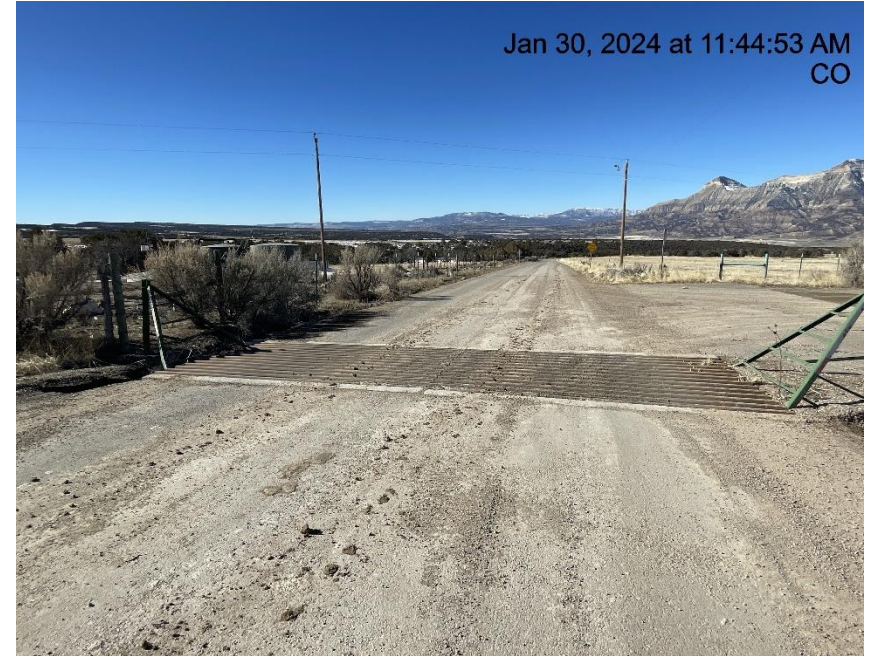
Photo # 4833 Insufficient tracking BMP's/tracking off location & onto to CR 306 (Spring Creek RD)
