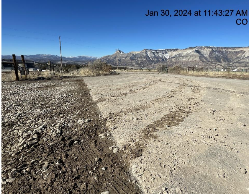
Photo # 4820 Insufficient tracking BMP's/tracking off location & onto to CR 306 (Spring Creek RD)
