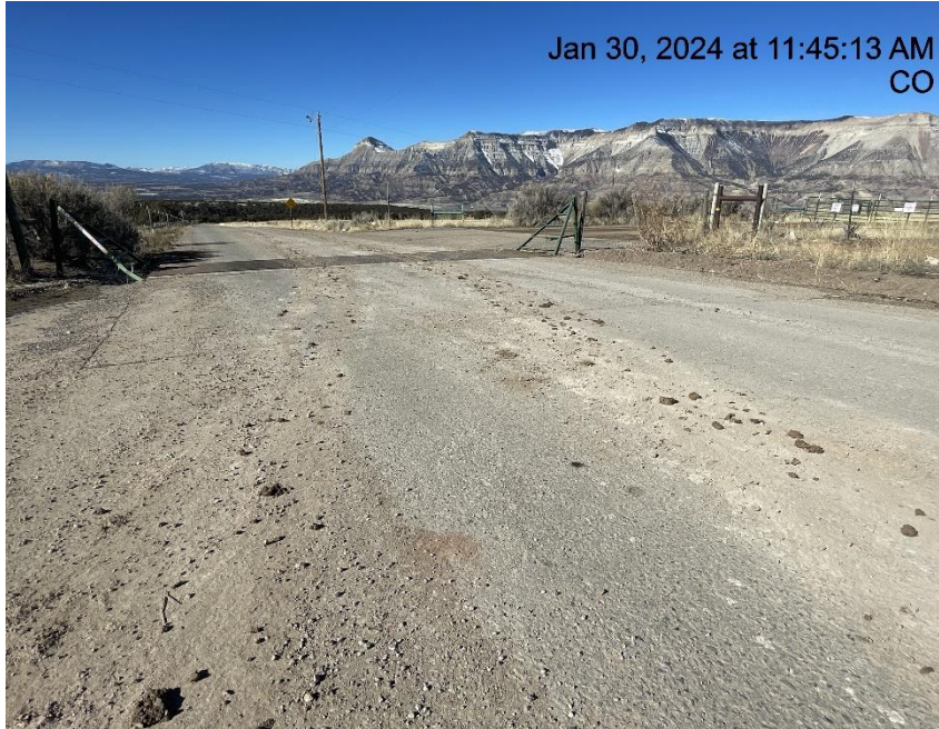
Photo # 4832 Insufficient tracking BMP's/tracking off location & onto to CR 306 (Spring Creek RD)
