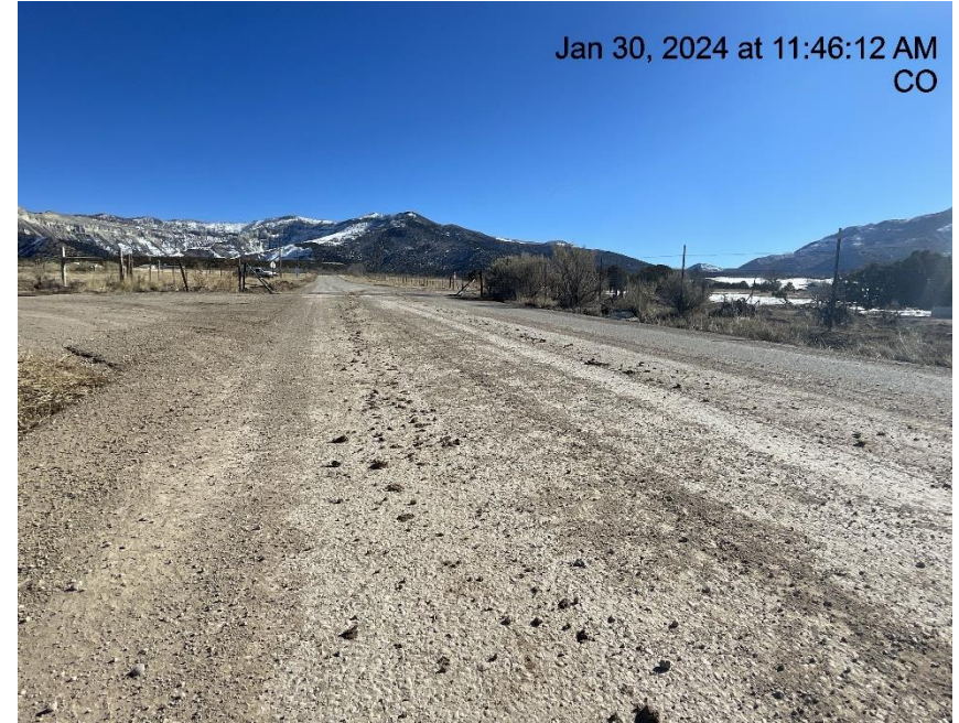
Photo # 4837 Insufficient tracking BMP's/tracking off location & onto to CR 306 (Spring Creek RD)
