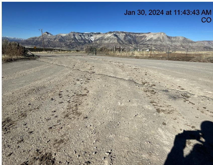
Photo # 4822 Insufficient tracking BMP's/tracking off location & onto to CR 306 (Spring Creek RD)
