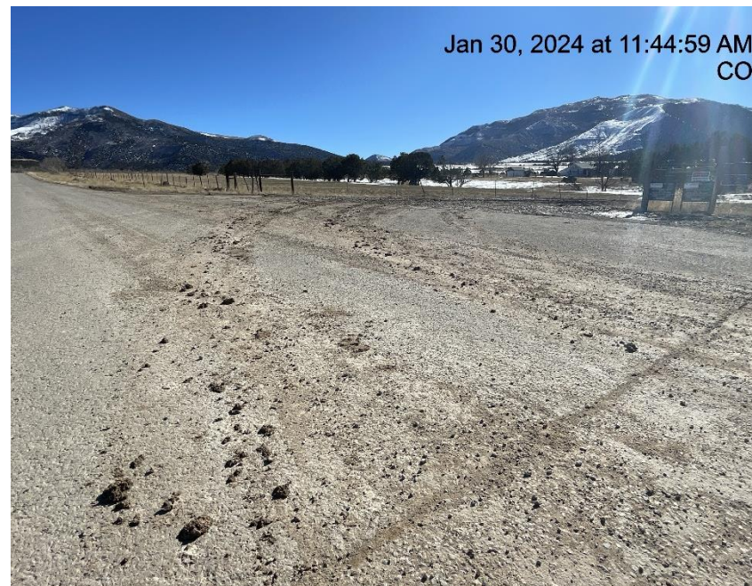
Photo # 4829 Insufficient tracking BMP's/tracking off location & onto to CR 306 (Spring Creek RD)
