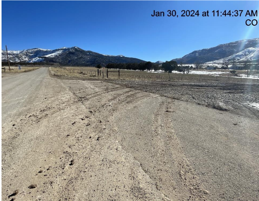
Photo # 4826 Insufficient tracking BMP's/tracking off location & onto to CR 306 (Spring Creek RD)
