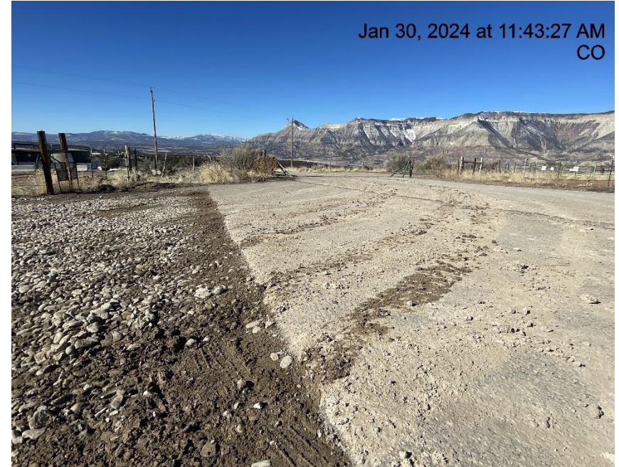
Photo # 4819 Insufficient tracking BMP's/tracking off location & onto to CR 306 (Spring Creek RD)
