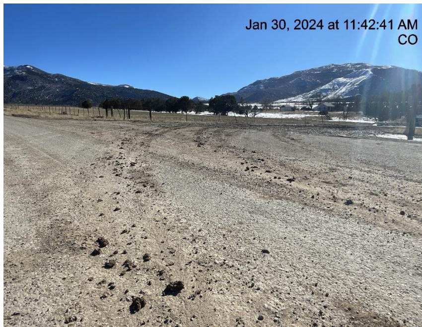
Photo # 4830 Insufficient tracking BMP's/tracking off location & onto to CR 306 (Spring Creek RD)
