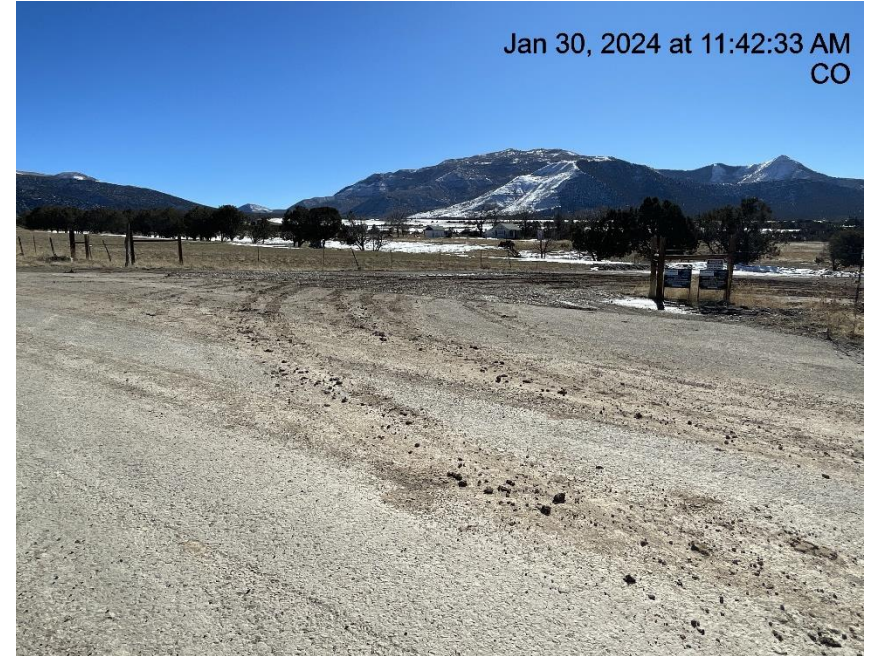
Photo # 4825 Insufficient tracking BMP's/tracking off location & onto to CR 306 (Spring Creek RD)
