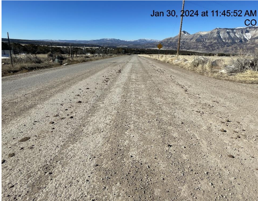
Photo # 4836 Insufficient tracking BMP's/tracking off location & onto to CR 306 (Spring Creek RD)
