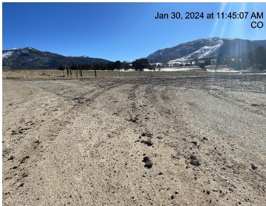
Photo # 4828 Insufficient tracking BMP's/tracking off location & onto to CR 306 (Spring Creek RD)
