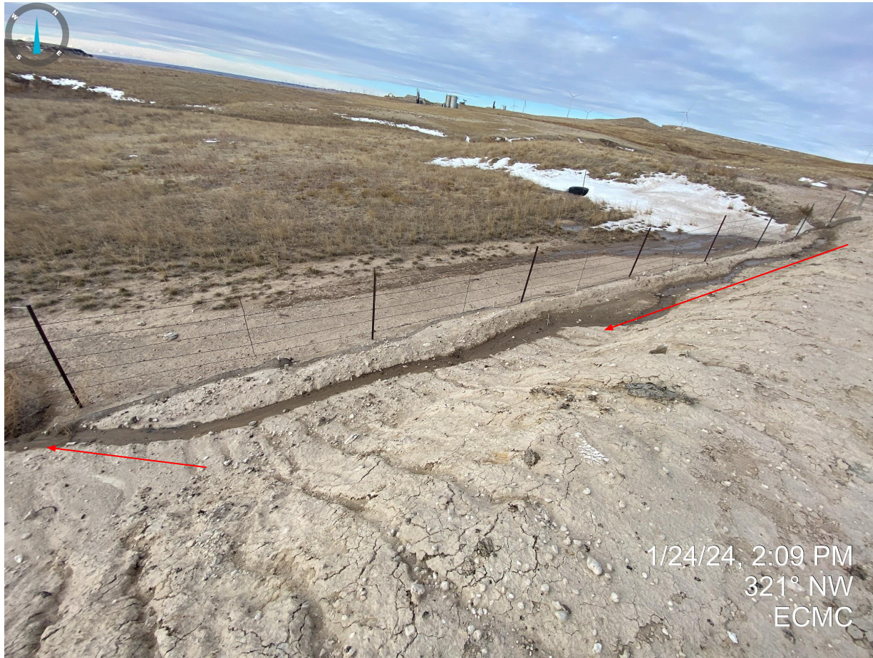
Photo 12. Taken near the southwest corner of the pit. During this inspection, Staff observed stormwater actively discharging off location into the adjacent salt kill areas. Stormwater control measures are inadequate for this location.
