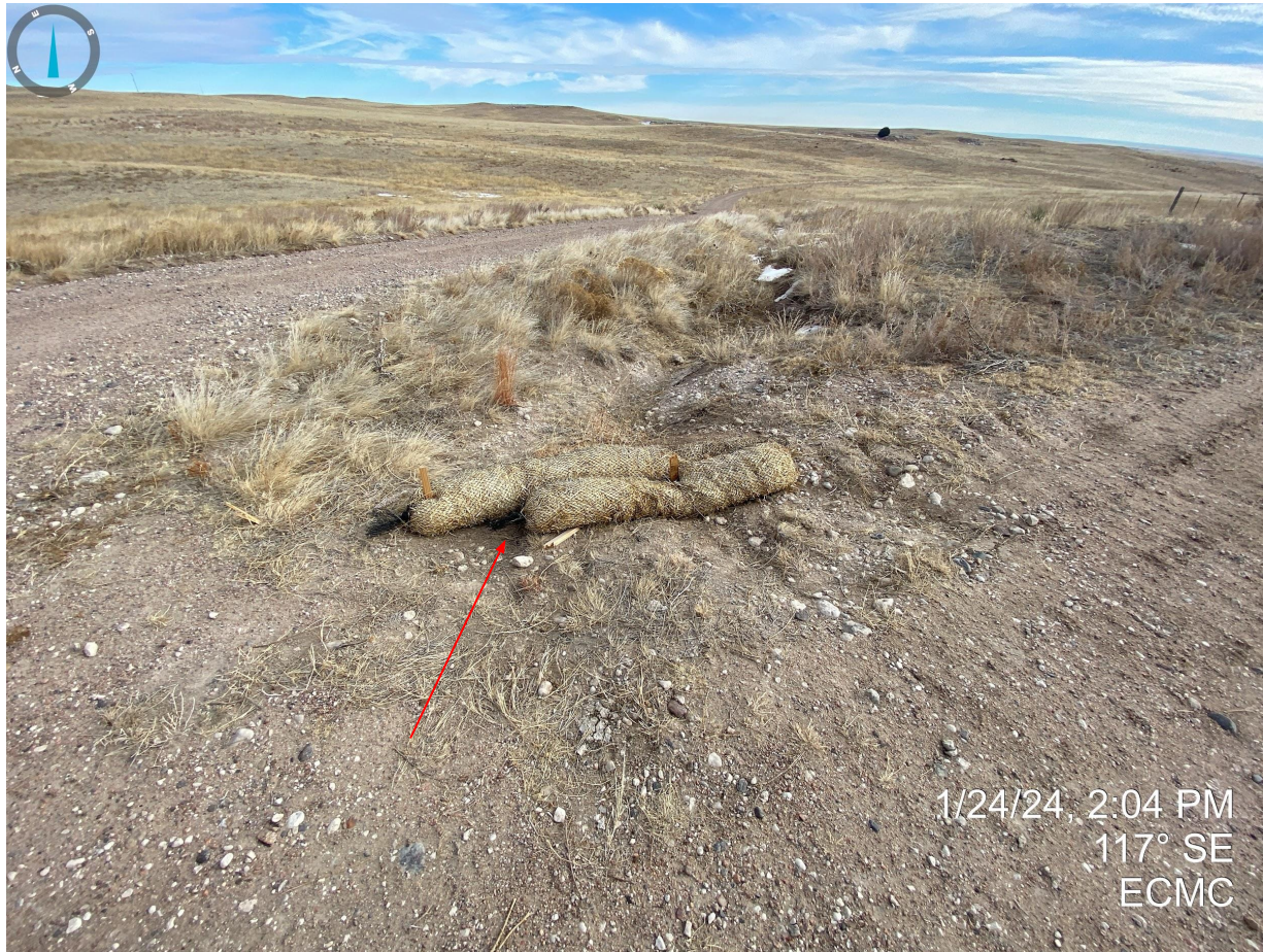
Photo 9. Stormwater control measures installed near the production areas/access road do not appear to be properly installed per good engineering practices (e.g. trenched and backfilled).
