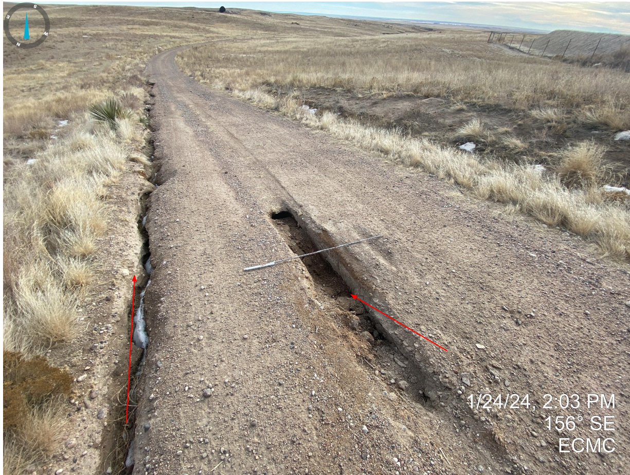
Photo 7. Subsidence observed along the access road. Also pictured, erosion degradation along the access road.
