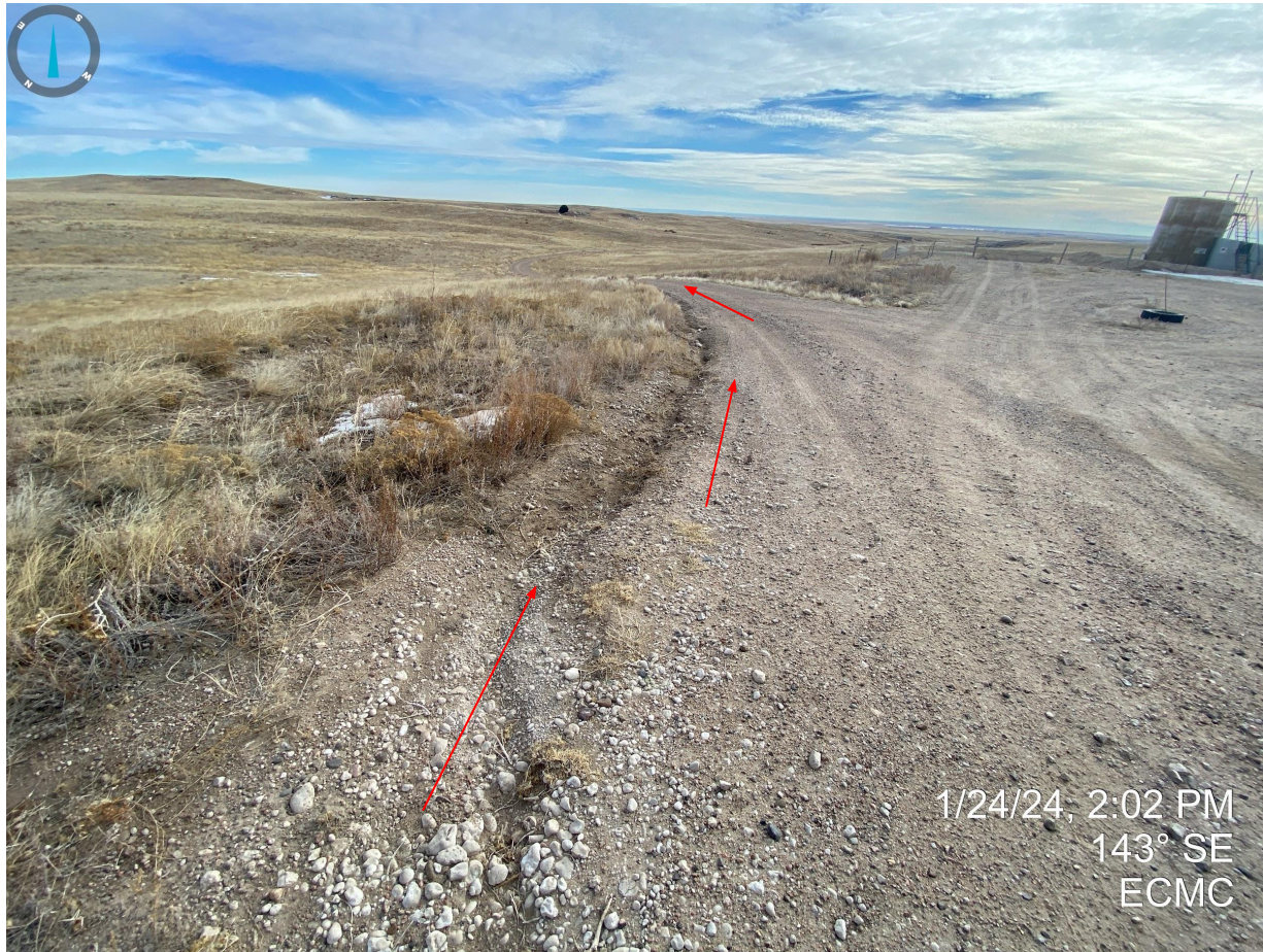
Photo 5. Taken from the access road east of the pit. Evidence of erosion degradation, previously documented, does not appear to have been repaired/stabilized with no evidence of control measures/BMPs observed that would prevent further erosion of the access road.
