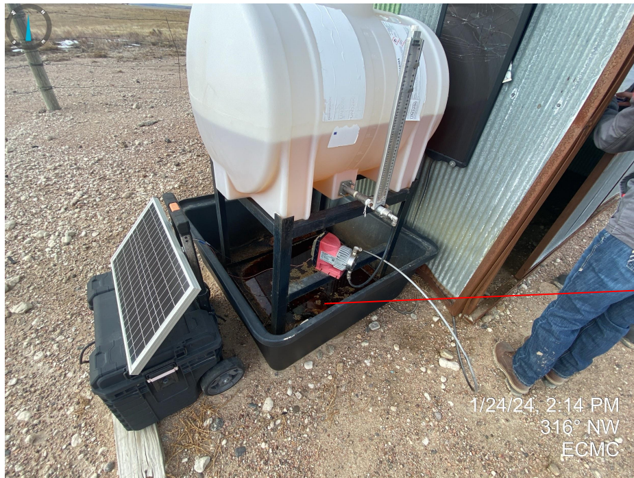
Photo 19. A wildlife mortality was observed within an uncovered secondary containment at the injection well day tank.
