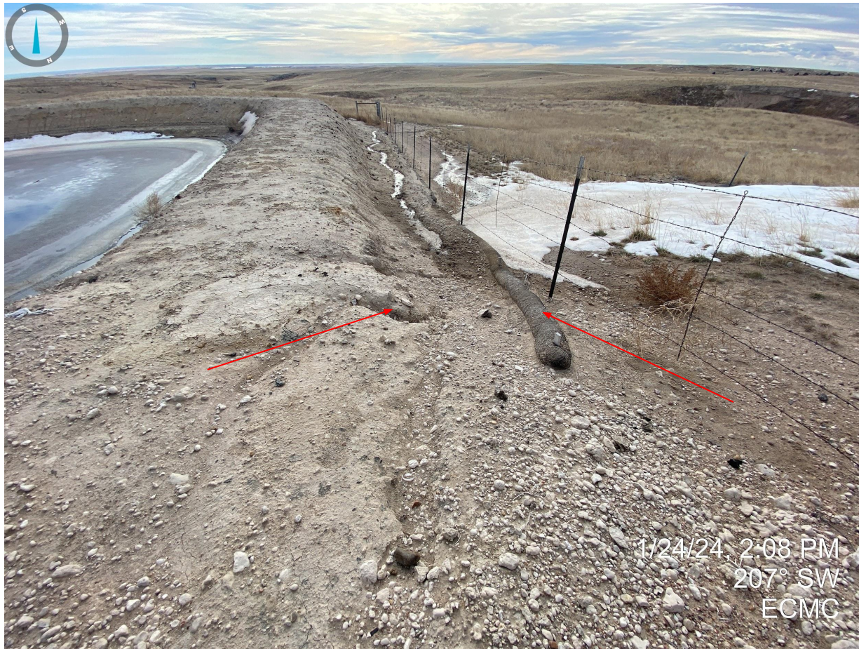
Photo 11. Taken from the northwestern portion of the pit. Photo illustrates erosion degradation on the pit walls and inadequate stormwater control measures around the base, or perimeter, of the pit.
