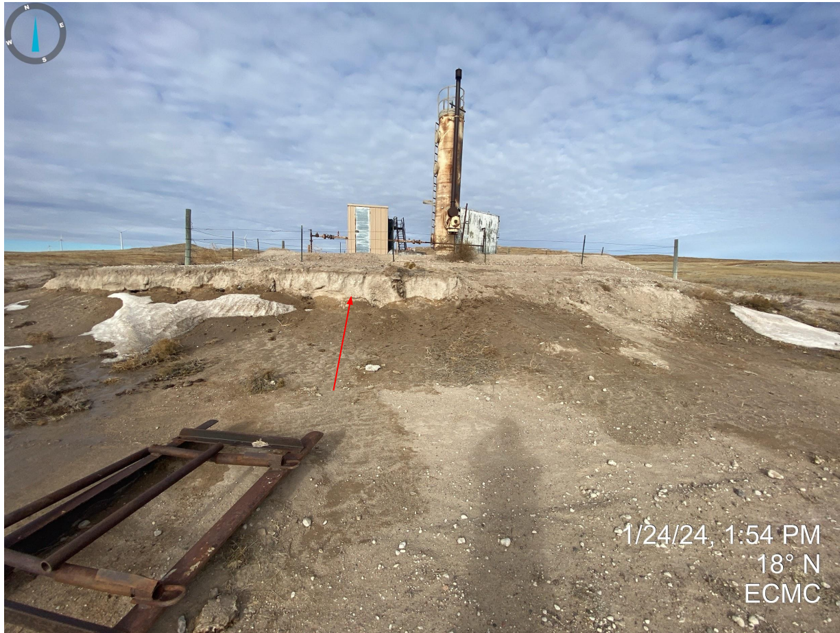
Photo 1. Taken near the vertical heater treater. Erosion degradation previously documented does not appear to have been repaired, and there is no evidence that stormwater control measures have been implemented to protect the unstabilized soils.
