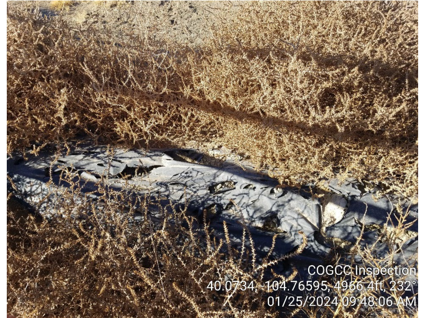
Photo 10 - Former E&P Waste area. Holes in lining.
