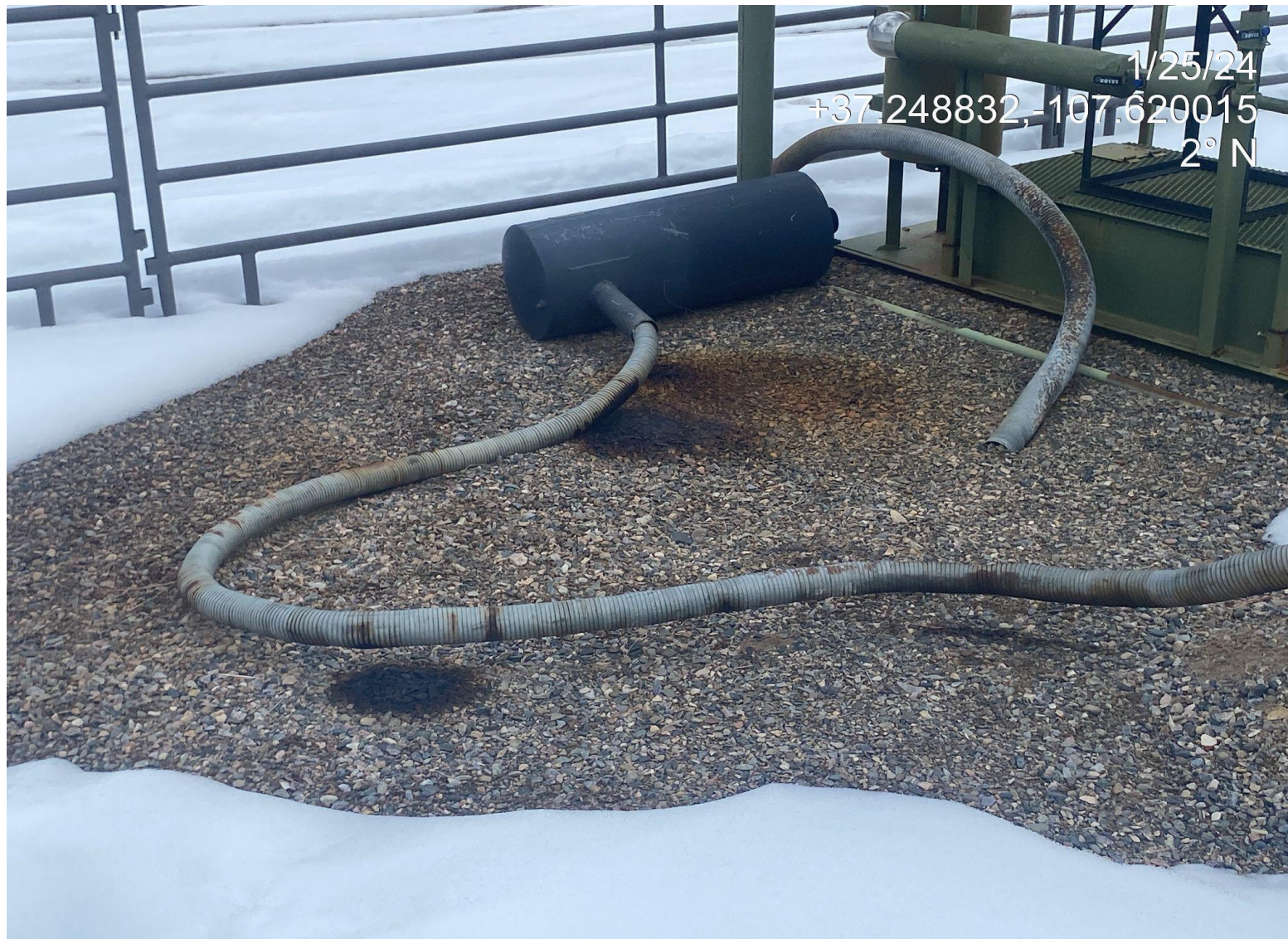
Photo 2. View of stained soil around muffler.
