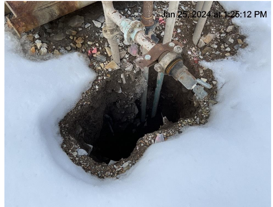
Photo # 4052 Hole in ground near sales gas meter house/safety issue/wildlife & personnel hazard
