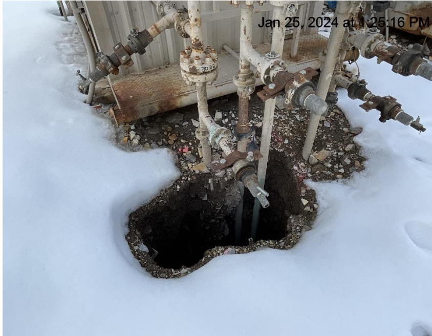
Photo # 4053 Hole in ground near sales gas meter house/safety issue/wildlife & personnel hazard
