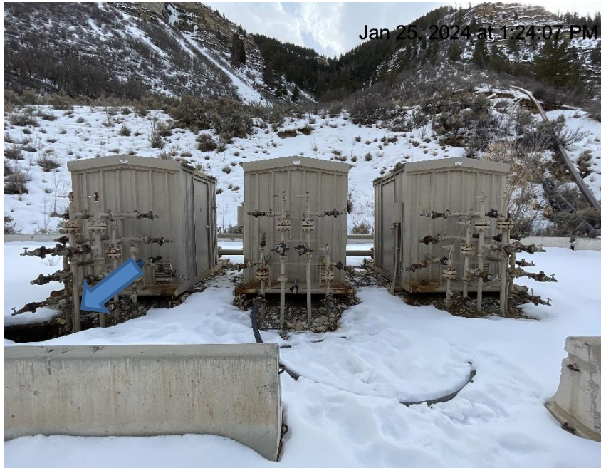
Photo # 4049 Hole in ground near sales gas meter house/safety issue/wildlife & personnel hazard
