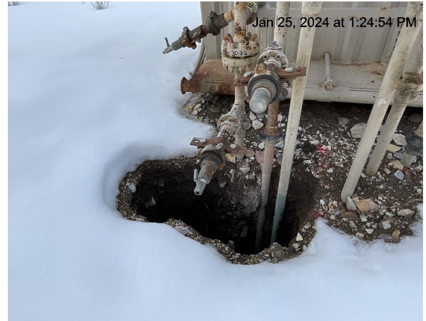
Photo # 4050 Hole in ground near sales gas meter house/safety issue/wildlife & personnel hazard
