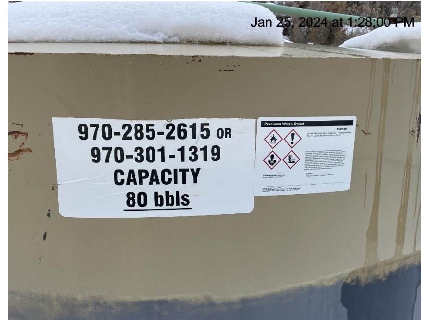
Photo # 4048 Labeling on blowdown tank missing required info & has inaccurate info
