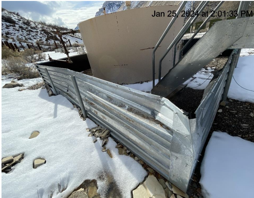
Photo # 4119 Tank containment damaged/buckling
