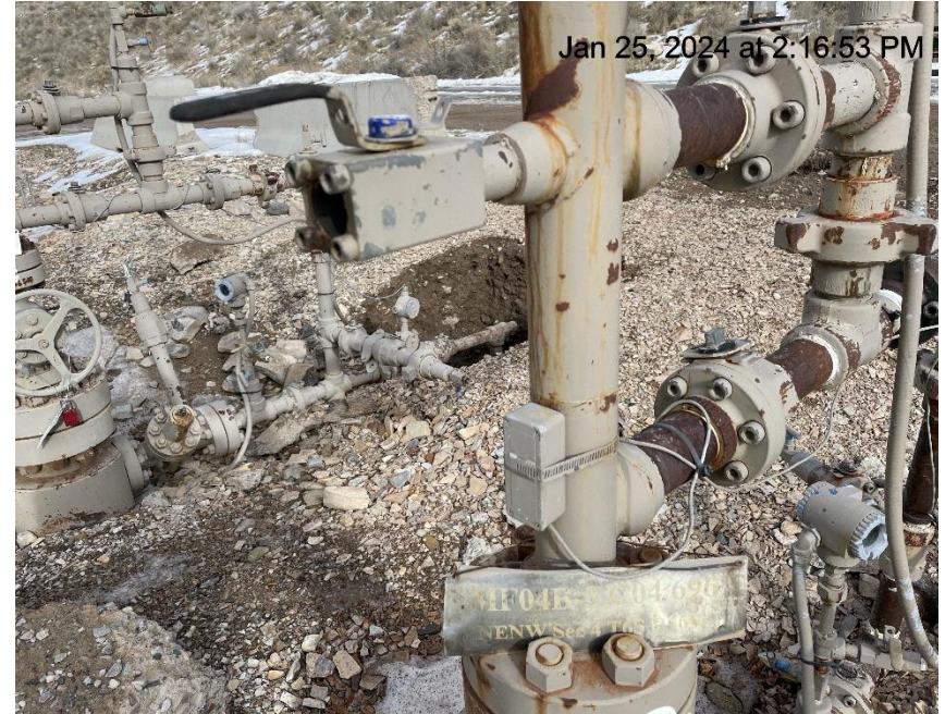
Photo # 4110 Open valve leaking gas on the MF04B-3 wellhead
