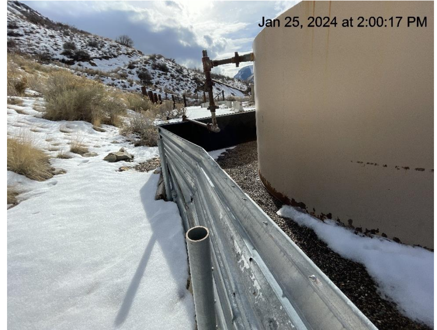
Photo # 4118 Tank containment damaged/buckling
