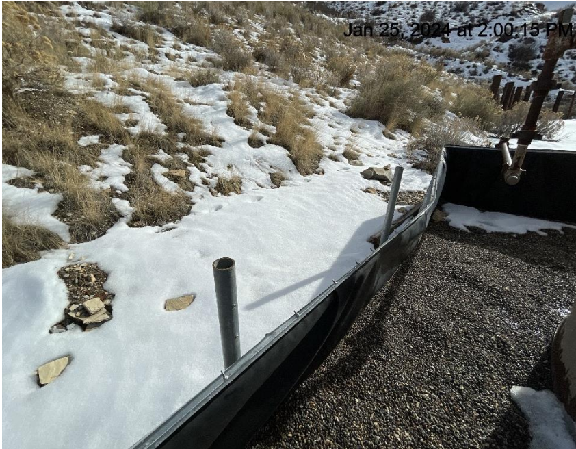
Photo # 4117 Tank containment damaged/buckling
