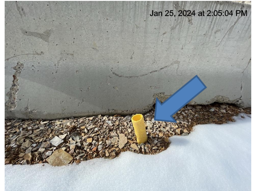
Photo # 4116 Improperly marked deadman
