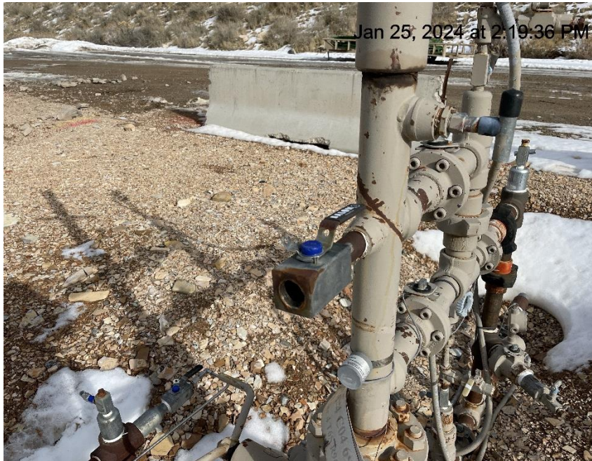
Photo # 4111 Open valve leaking gas on the MF07A-4 wellhead
