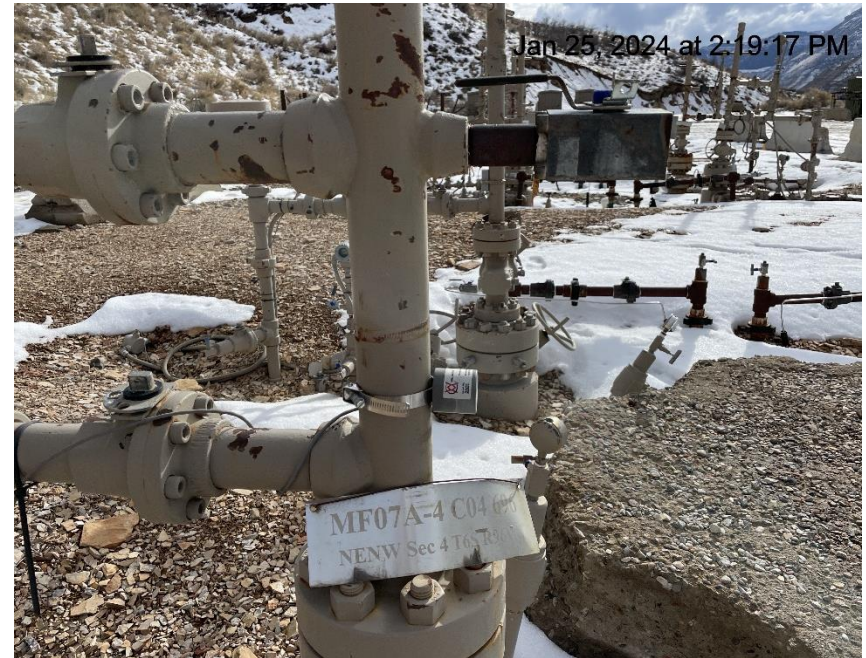
Photo # 4112 Open valve leaking gas on the MF07A-4 wellhead
