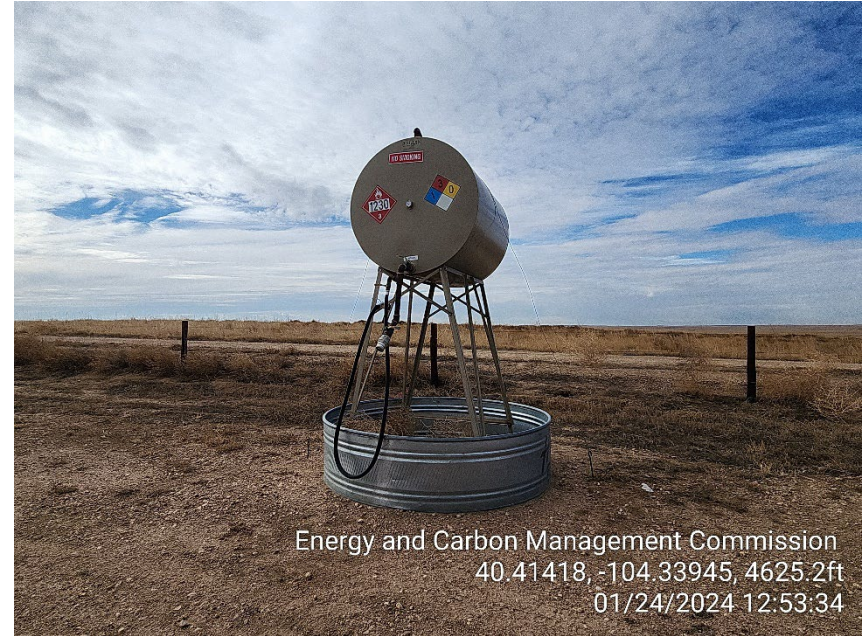
Photo 2 – Methanol Day Tank at Entrance – Tumbleweed Debris and Wildlife Netting
