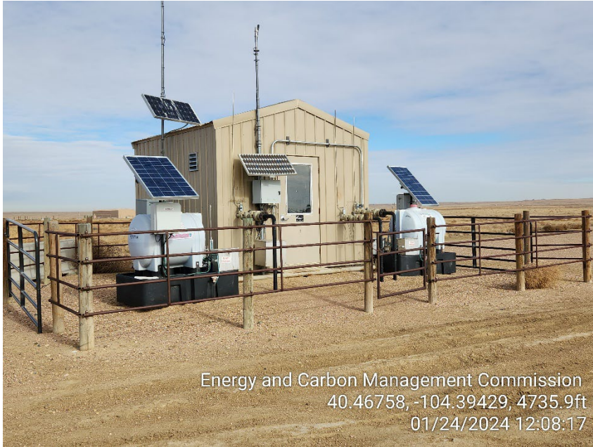
Photo 1 – West Gas Lift Injection Meter House
