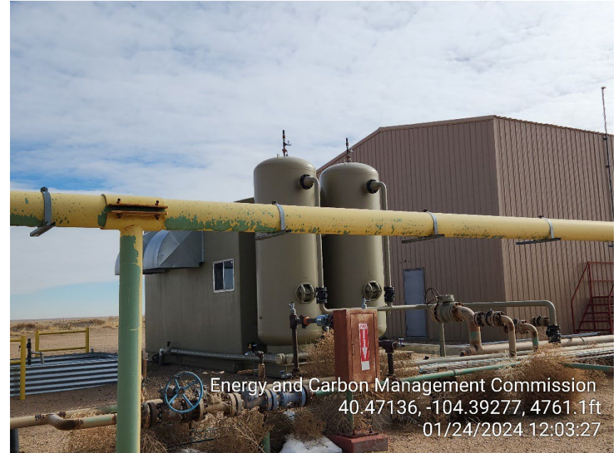
Photo 14 – Instrumental Air Unit
