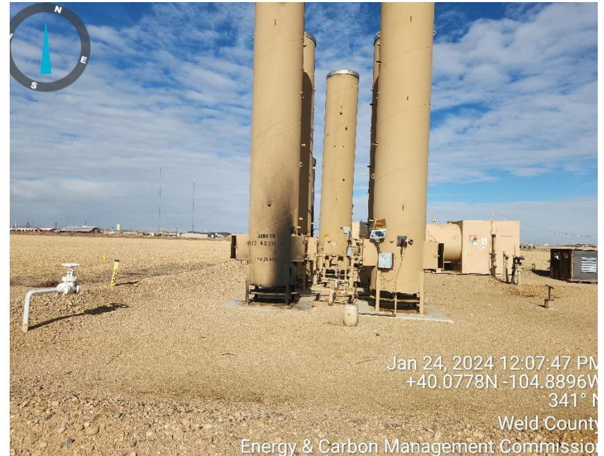
Photo 6 out of service ECD due to fire
