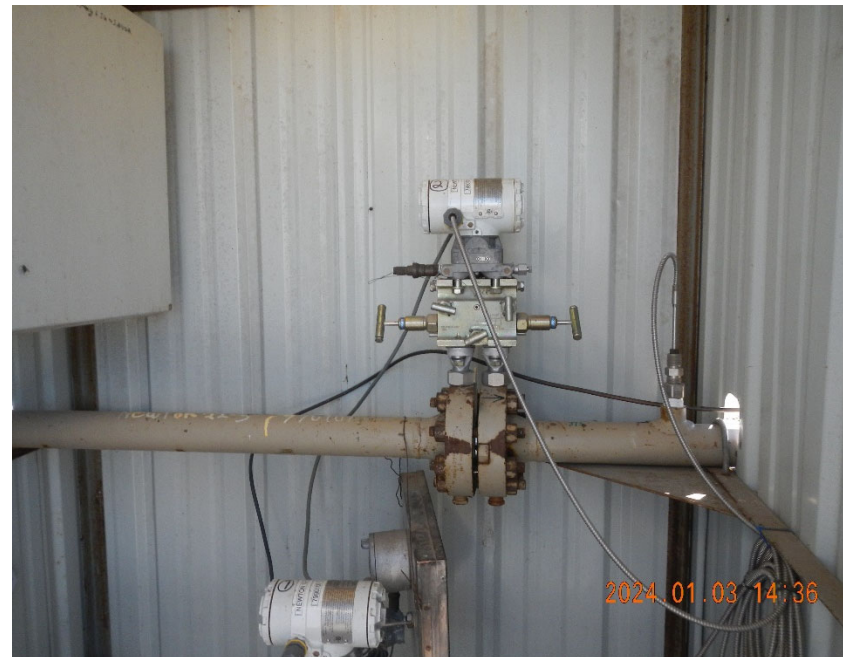
8. Digital gas meter inside shared meter shed.
