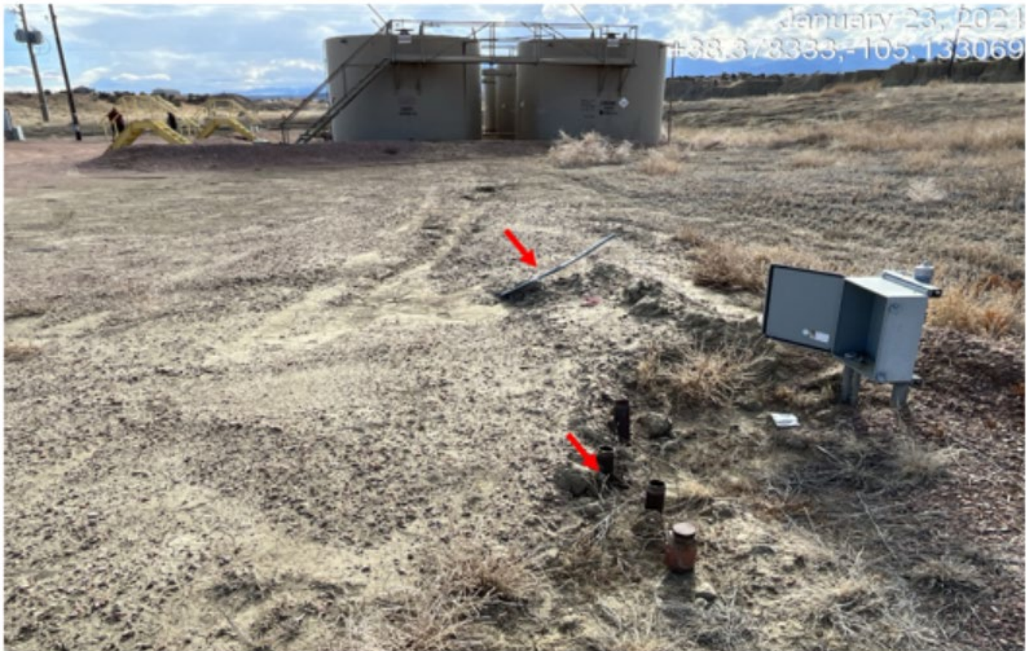
Photo 4. Facing south at the west side of the location. There is an exposed electric line at red arrow and multiple open pipe risers. All risers and utilities need to be removed. Previous corrective action was not completed.
