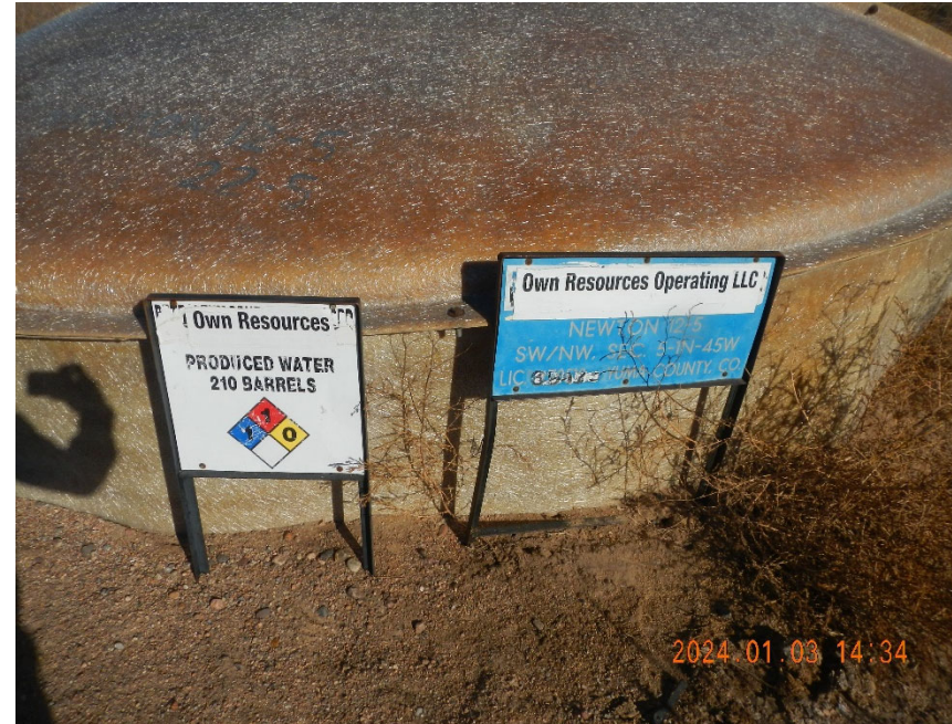
8. Signs at produced water tank. No contact information posted.
