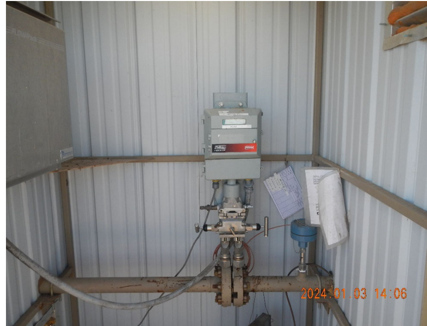
6. Digital gas meter inside meter shed.
