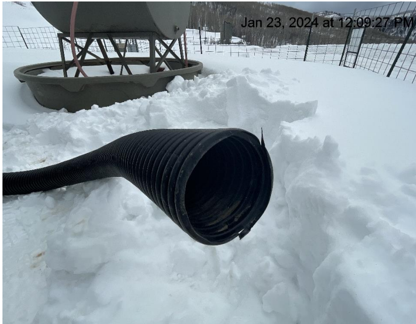
Photo # 3550 Flowline heating insulation open ended/wildlife hazard/available for entry by wildlife
