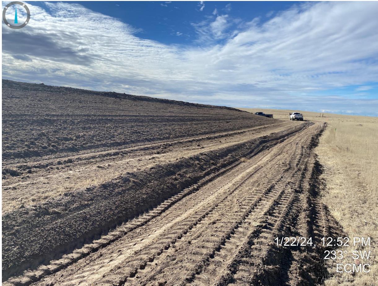
Photo 16. Taken on the northern portion of the location, near the topsoil stockpile. Perimeter ditch and berm observed.
