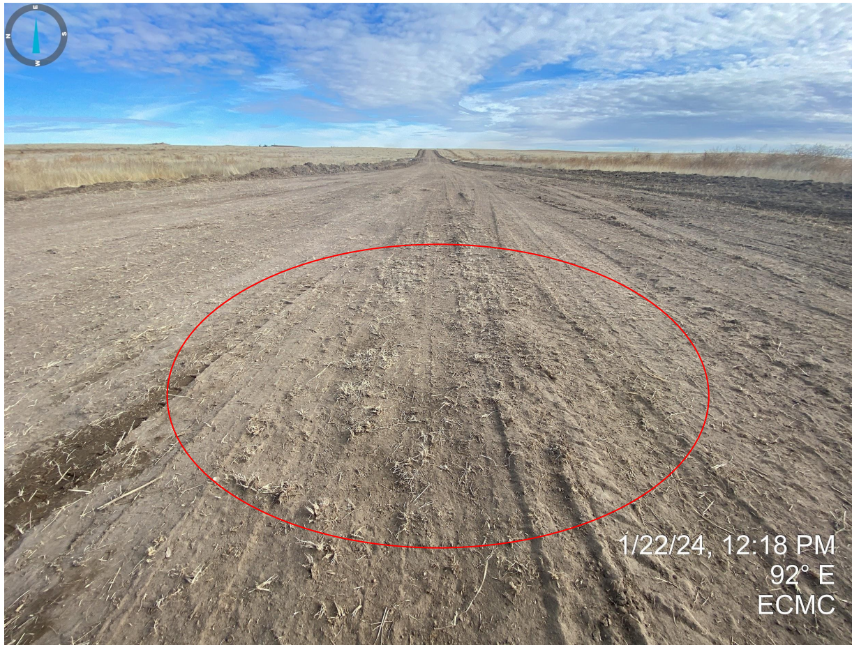
Photo 1. Taken from the location entrance, west side of the new access road. It doesn't appear that all topsoil has been salvaged from the access road with the presence of organic matter seen in the photo.
