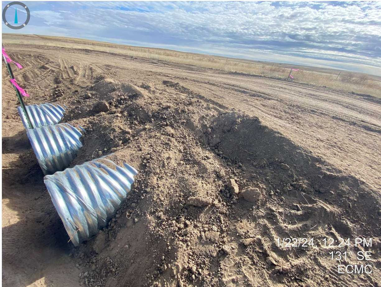
Photo 7. Taken at the eastern culvert crossing. It appears that topsoil has been used as fill material at one of the culvert crossings.
