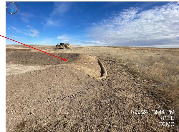
Photo 13. Sediment trap located on the southern portion of the location; temporarily stabilized inlet/outlet BMPs.
