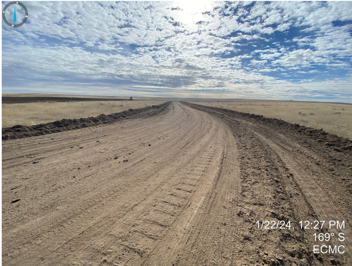
Photo 9. Taken near the location entrance, facing south along the new access road. It doesn't appear that all topsoil has been salvaged from the access road.
