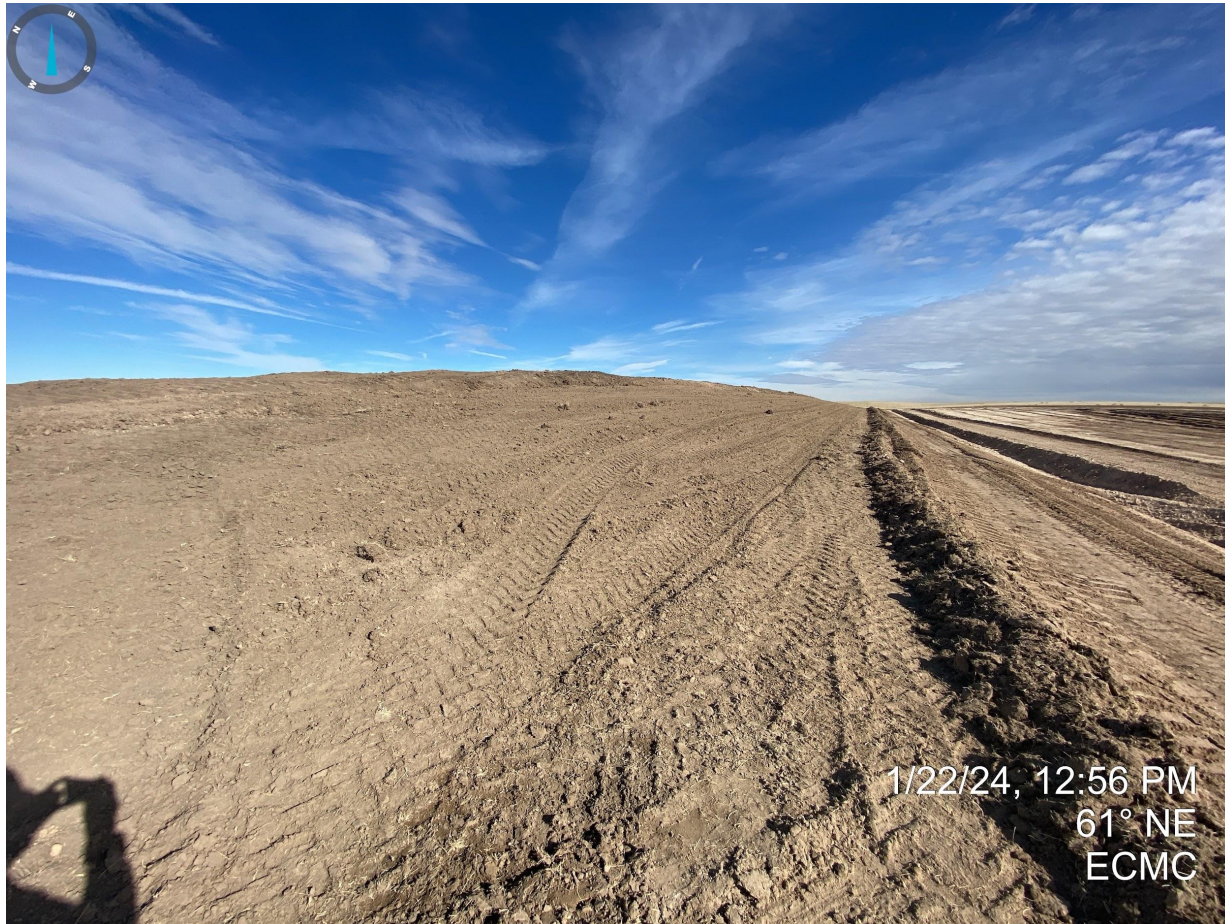
Photo 17. Taken from the southwest corner of the topsoil stockpile. It appears that topsoil from the drilling area has been stockpiled on the northern portion of the pad. Construction activities are ongoing and the Operator shall ensure that all stockpiled soils are temporarily stabilized (e.g. tracking, tackifier, etc) to prevent wind and water erosion degradation.
