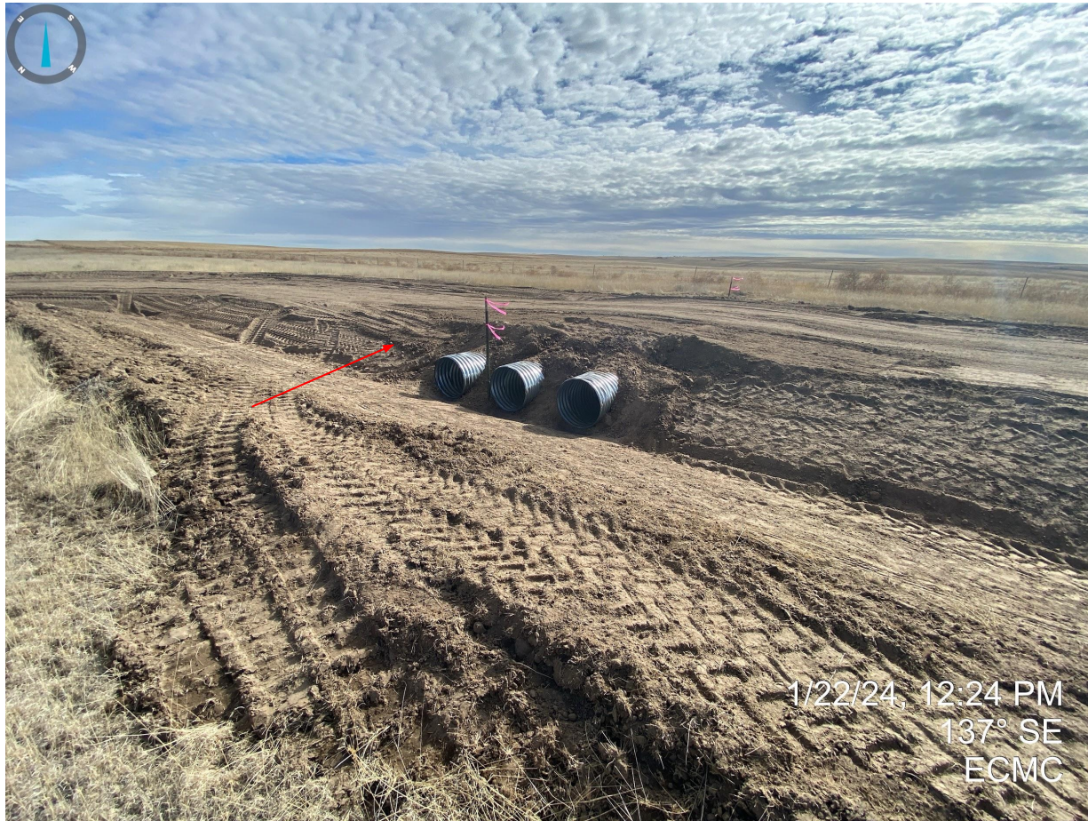
Photo 6. Taken at the eastern culvert crossing. It appears that topsoil has been used as fill material at one of the culvert crossings. Stormwater BMPs are still in process as construction activities are ongoing.
