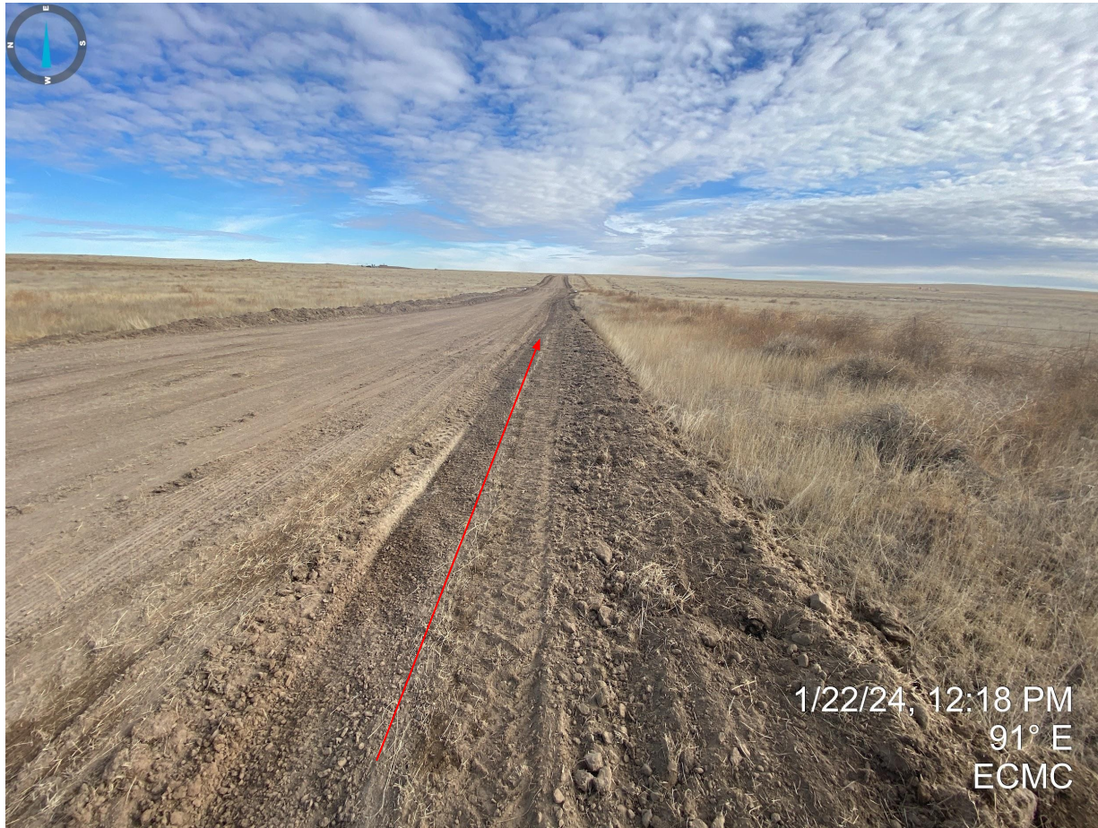
Photo 2. Taken from the western portion of the access road, near the entrance. A ditch and berm has been constructed, however the berm material is not consolidated and requires additional BMPs to protect from wind and water erosion.
