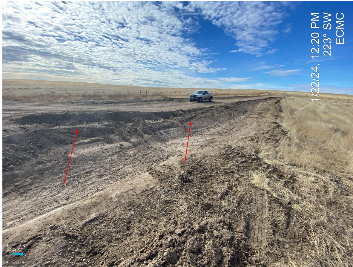
Photo 4. Taken at the western culvert crossing. It appears that topsoil has been used as fill material at one of the culvert crossings.
