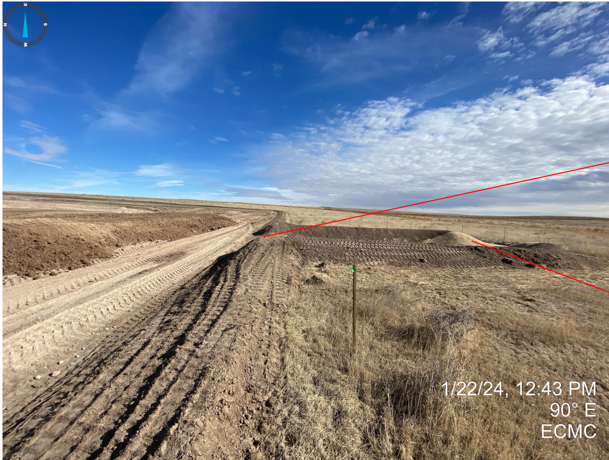
Photo 13. Sediment trap located on the southern portion of the location; temporarily stabilized inlet/outlet BMPs.
