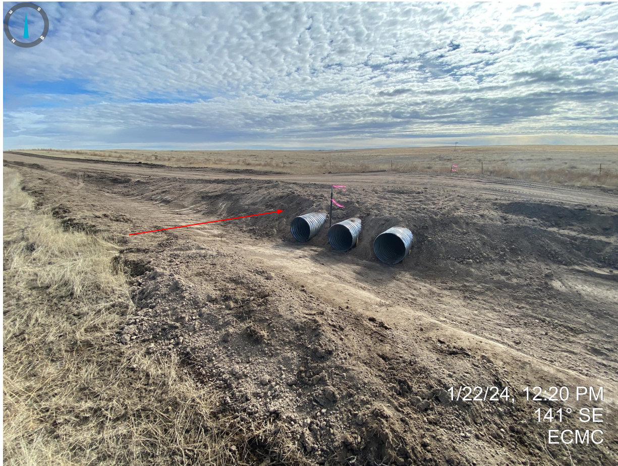
Photo 3. Taken from the access road. It appears that topsoil has been used as fill material at one of the culvert crossings. Stormwater BMPs are still in process as construction activities are ongoing.
