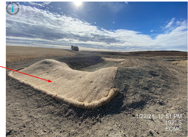
Photo 15. Sediment trap located on the northeast corner of the location; temporarily stabilized inlet/outlet BMPs.
