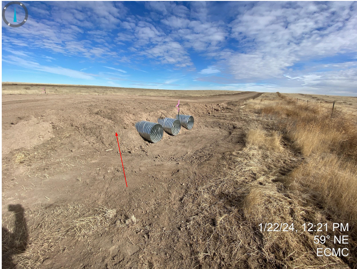
Photo 5. Taken at the western culvert crossing. It appears that topsoil has been used as fill material at one of the culvert crossings.
