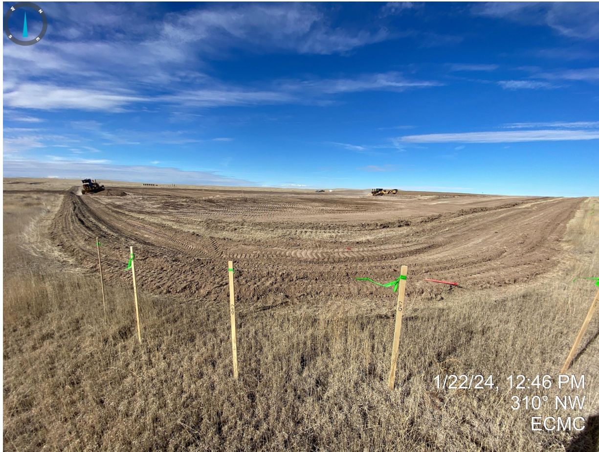
Photo 14. Taken from the southeast corner of the location. Perimeter ditch and berm has been constructed around the construction area.
