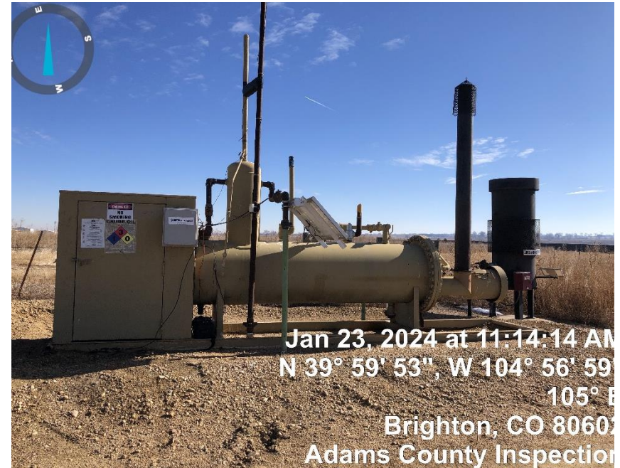
Photo#2 Separator/ECD/Automation RTU
