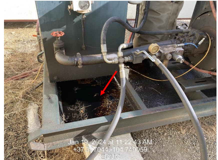
Photo 4 – Oily water in Engine Skid
