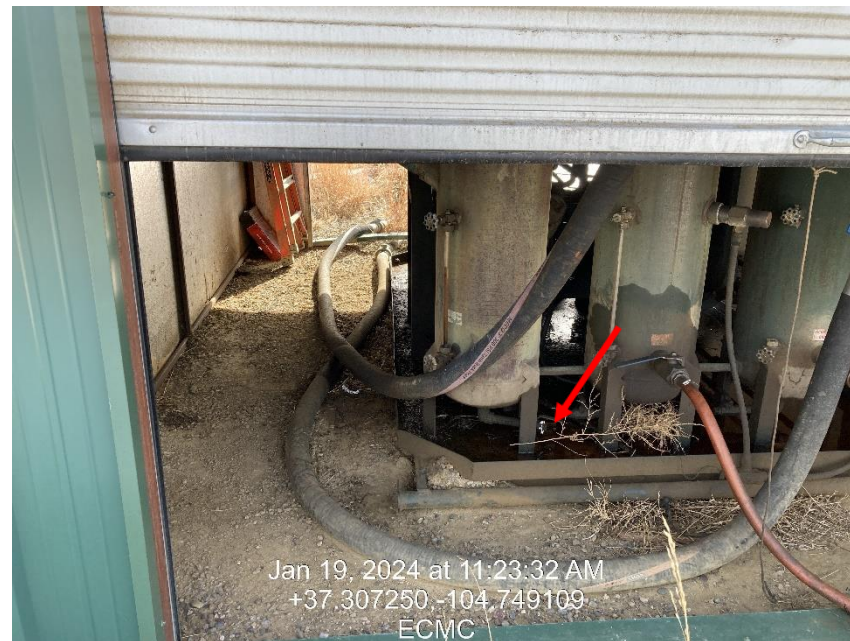
Photo 6 – Compressor in Building. Oil water in Skid
