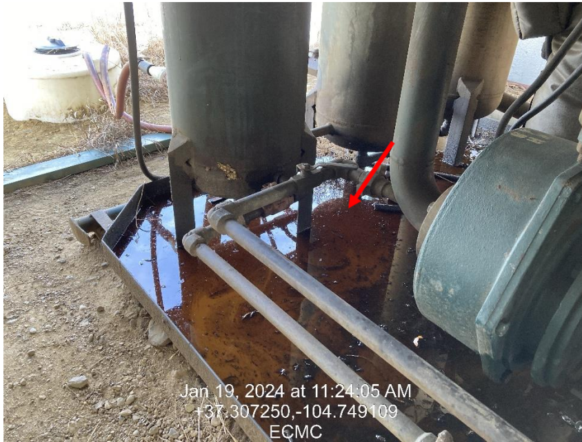
Photo 7 – Compressor in Building. Oil water in Skid
