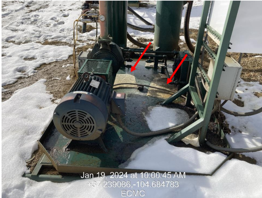
Photo 9 – Electric Compressor with oil diapers in skid pan.
