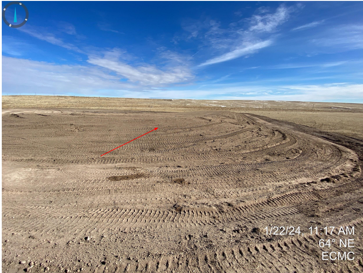
Photo 7. Taken from the western side of the topsoil stockpile. Staff estimates the topsoil stockpile is approximately 4,000 CY, which differs from the Operator submitted Topsoil Protection Plan estimates of 5,557 CY. Additionally, the topsoil stockpile requires temporary stabilization (e.g. equipment tracking, tackifiers, etc) to protect soils; construction activities were ongoing at the time of this inspection.
