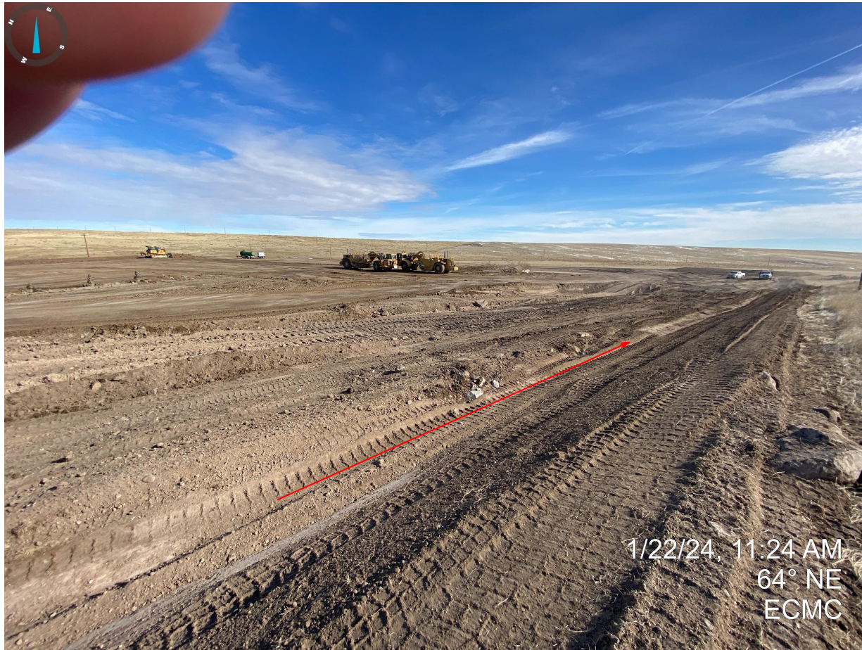
Photo 10. Taken near the southwest corner of the location. Photo illustrates perimeter ditch and berm.
