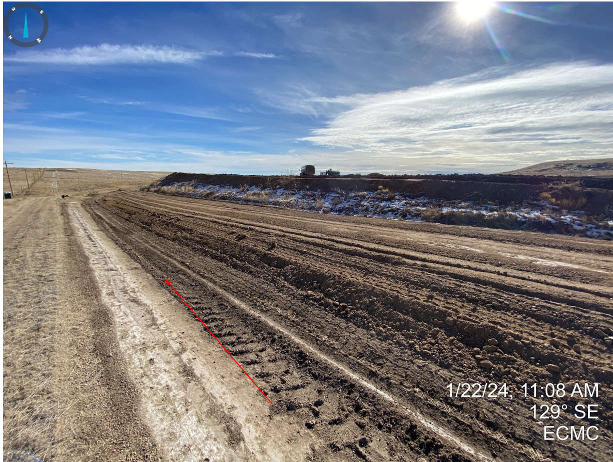
Photo 2. Northern portion of the construction area. Stormwater ditch has been installed around the perimeter of the disturbance area.
