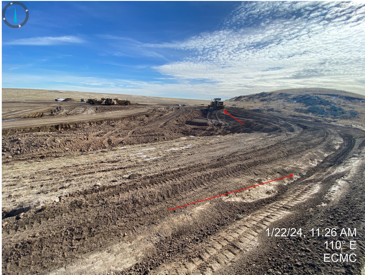
Photo 11. Taken from the western portion of the location. Photo illustrates crew using road grader to compact/wheel pack the perimeter ditch and berm BMPs.
