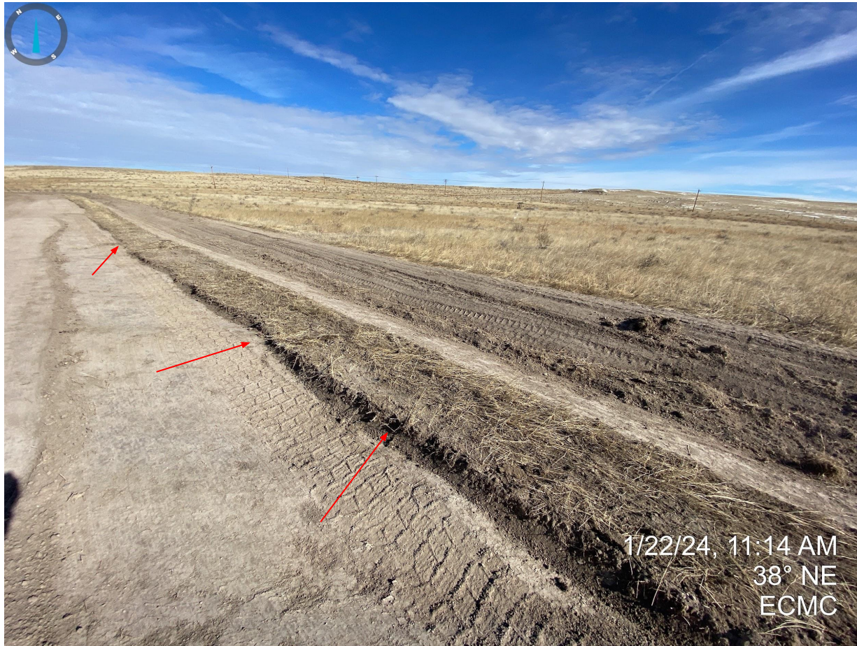
Photo 6. Taken from the east side of the location. Photo illustrates cut from topsoil salvage operations; the visible cut of the undisturbed topsoil vs the salvage area varied in depths of 3-6”.
