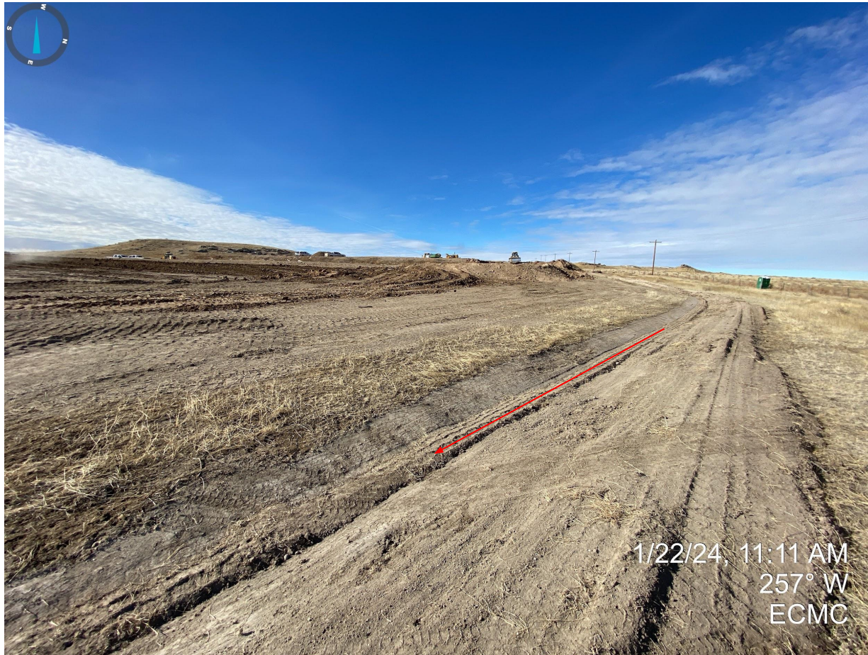
Photo 3. Northeastern portion of the construction area. Stormwater ditch has been installed around the perimeter of the disturbance area.
