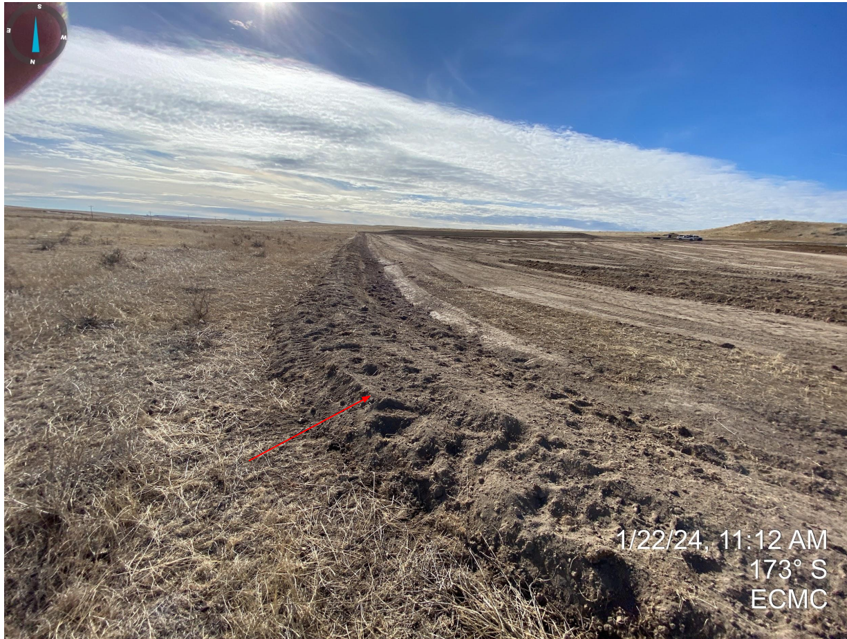
Photo 4. Northeastern portion of the construction area. Perimeter berm material is unconsolidated and requires BMPs to stabilize the soils. At the time of this inspection, Staff observed a road grader wheel packing the berm on the western side of the location; the Operator shall ensure all soils are adequately stabilized.
