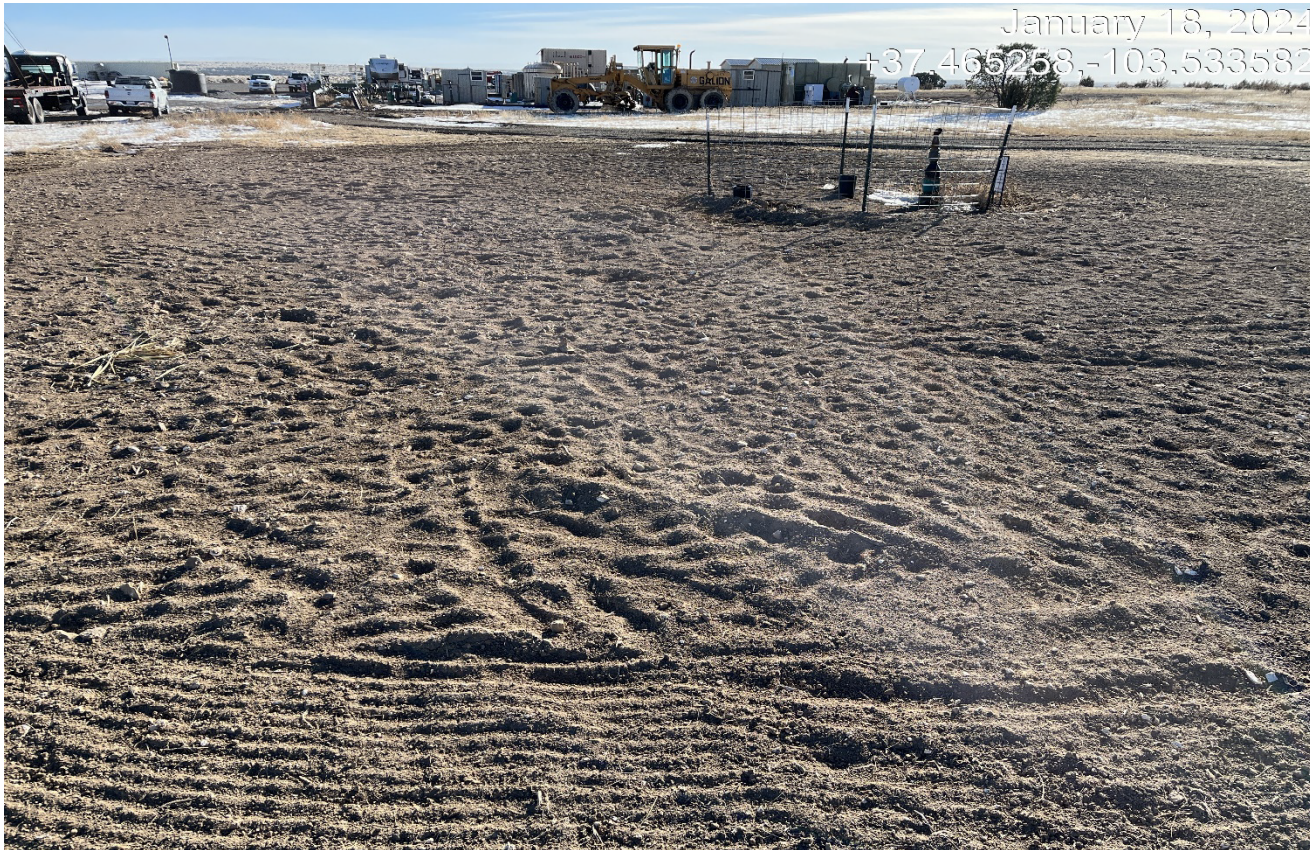
Photo 7. Facing south at the location. The excavated area at the wellhead has been backfilled and the rock debris has been removed. It is unknown what topsoil material was replaced since it was not properly salvaged. It does not appear soil closer to the well were seeded.
