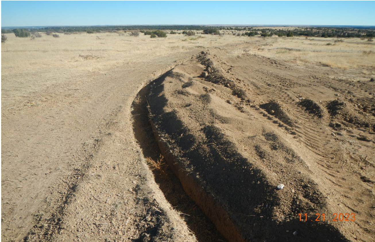
Photo 6. Facing east toward the flowline disturbance. Loose soils are susceptible to erosion and need to be stabilized.
