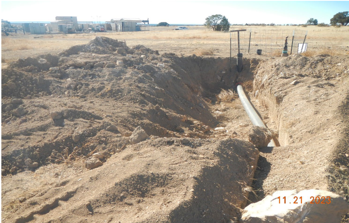
Photo 5. There is an open excavation at the wellhead and topsoil was not salvaged and protected. The open excavation at the wellhead and flowlineshow be properly marked/fenced to prevent livestock/wildlife entry.
