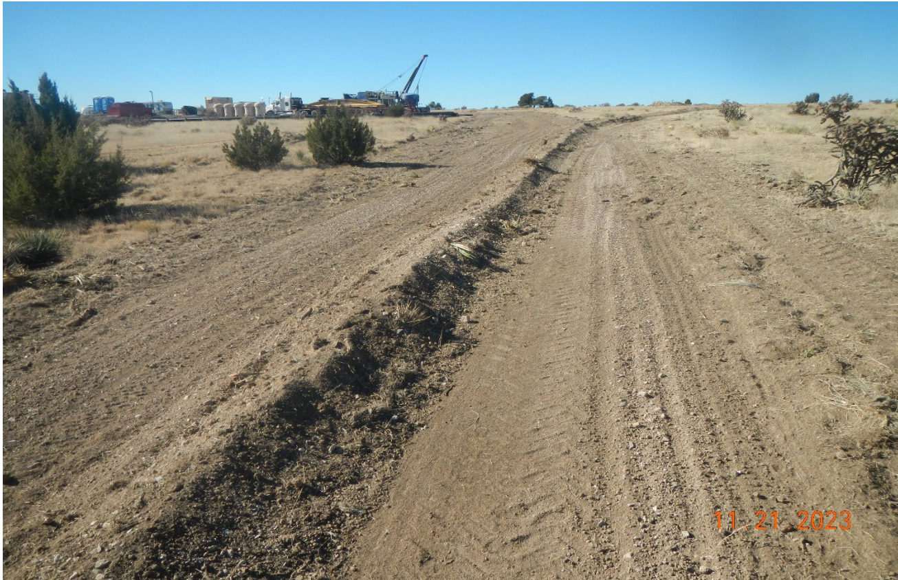
Photo 7. Standing further east of the location facing west along the flowline. Loose soils are susceptible to erosion and need to be stabilized.
