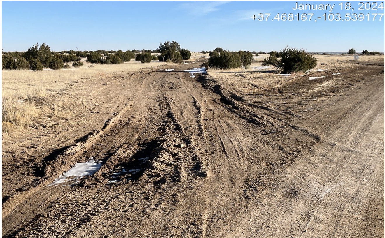
Photo 1. Facing southeast toward the access road to the Red Rocks #1-13 drill site. There is some signs rutting occurring onto the County Road.
