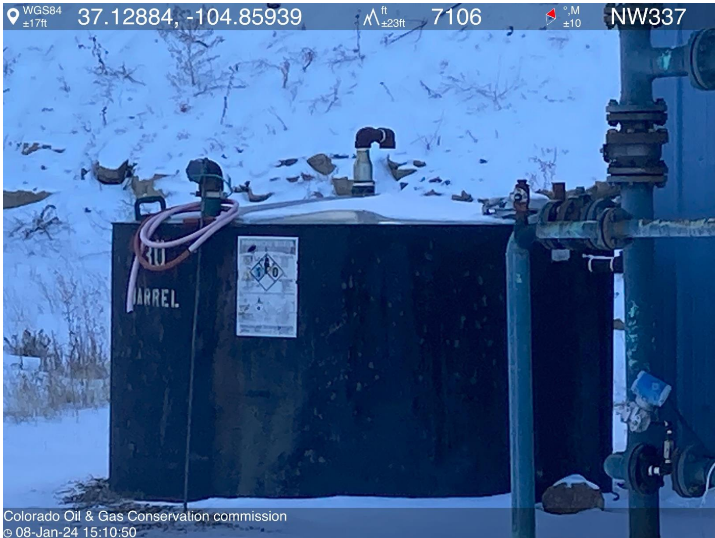
PHOTO 5: PRODUCED WATER TANK BATTERY.
