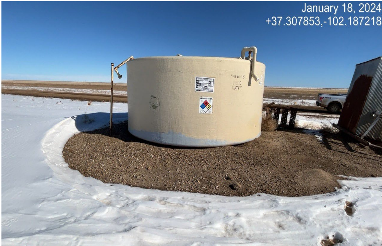
Photo 2. Facing toward the tank. There is not secondary containment at the tank.
