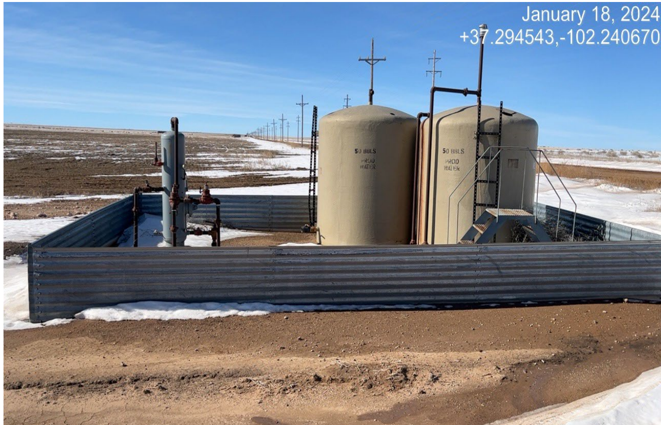
Photo 2. Facing toward the tanks with steel containment.
