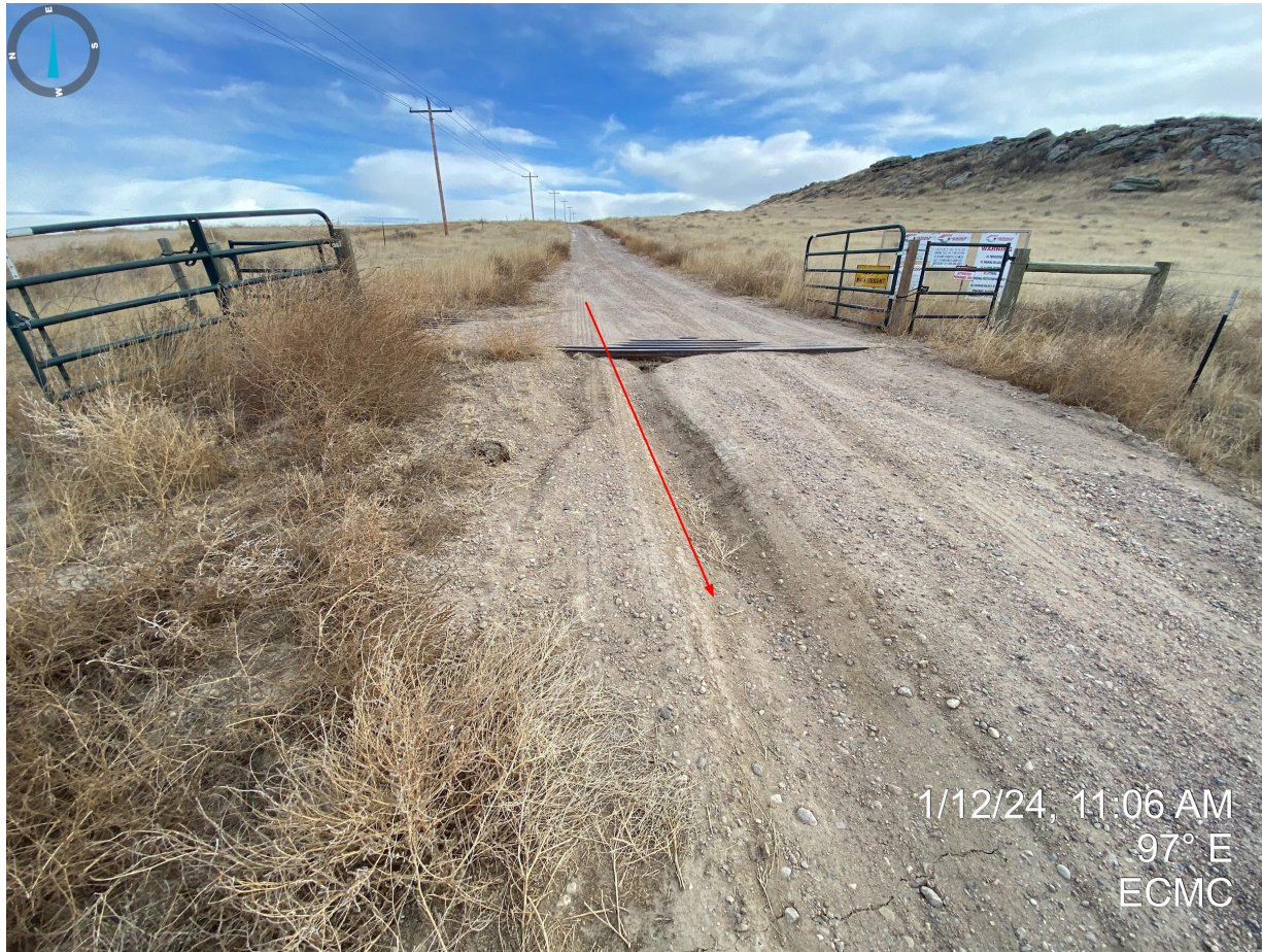
Photo 2. Erosion degradation at cattle guard.
