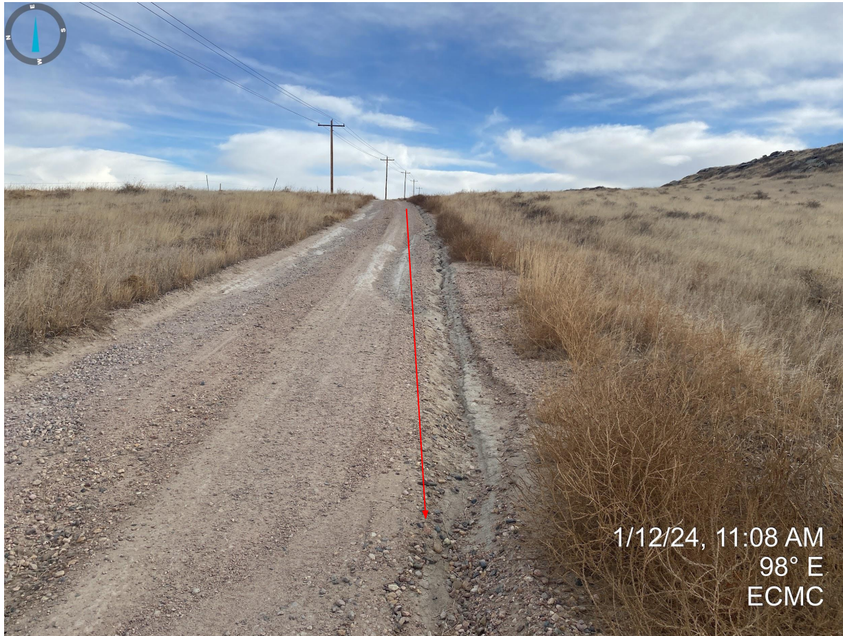
Photo 3. Erosion degradation and undesirable vegetation along the access road.
