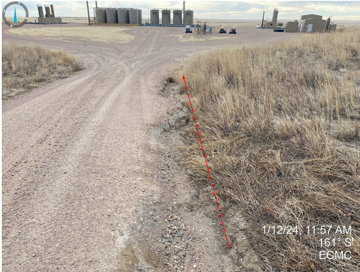
Photo 18. Gully erosion occurring on the access road leading to the production areas.
