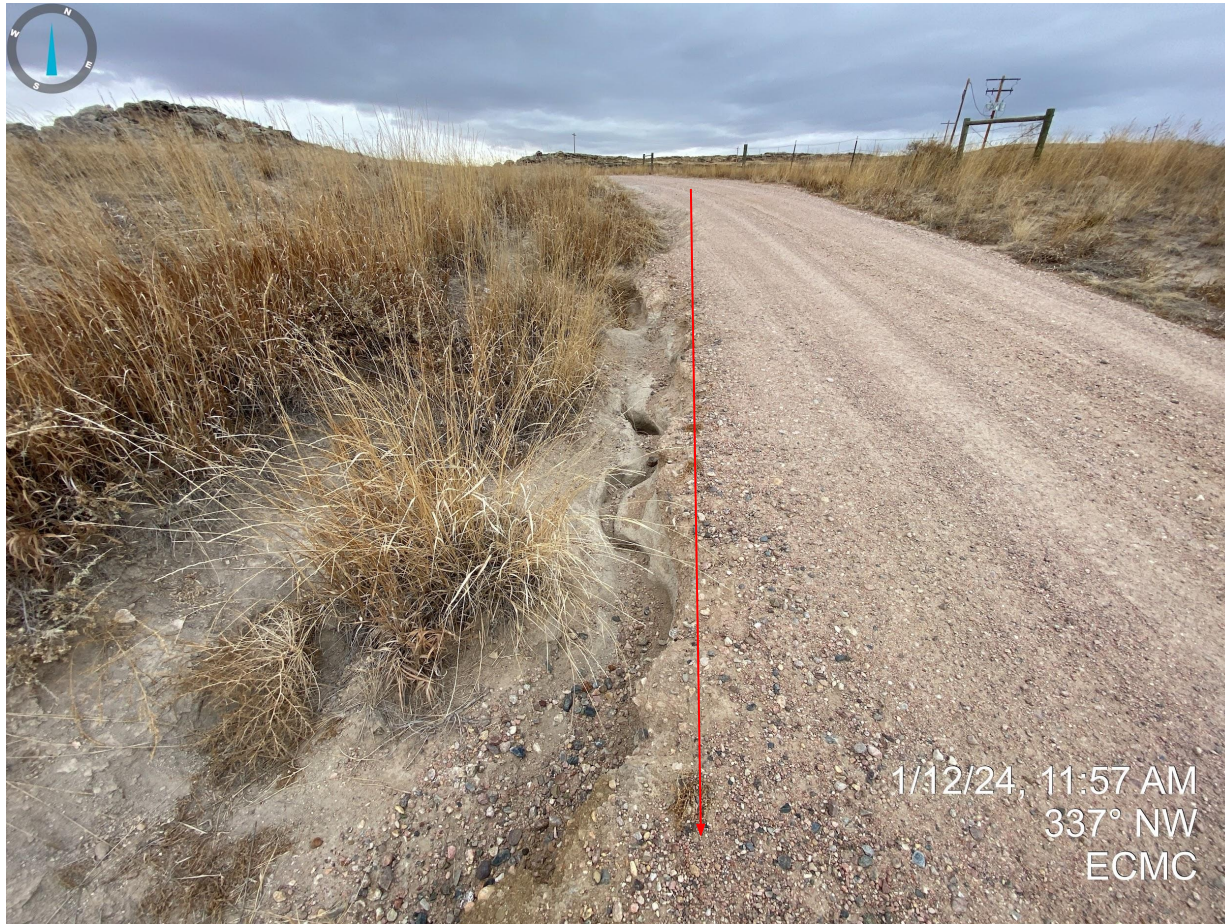
Photo 17. Gully erosion occurring on the access road leading to the production areas.
