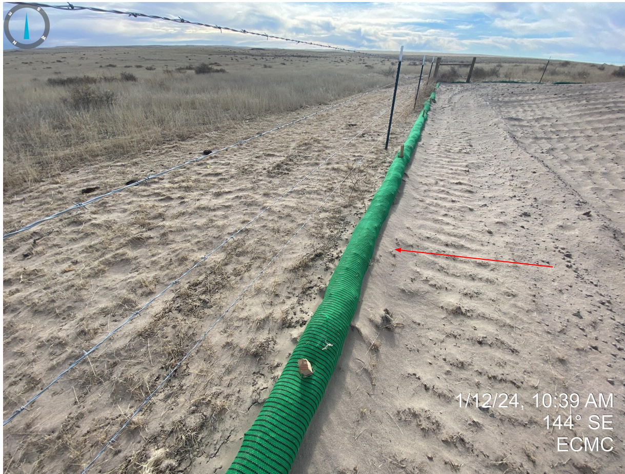
Photo 11. Filtrex requires maintenance as they're beginning to fill with soil.
