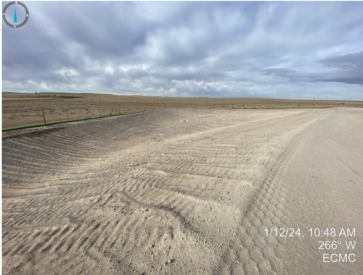
Photo 22. Southwest stormwater retention area. Stormwater controls have been equipment tracked, however, tracks are beginning to fill with soil which indicates additional stabilization BMPs are required (e.g. seeding, tackifiers, etc). The retention areas also do not appear to have any protected/armored inlet or outlets.
