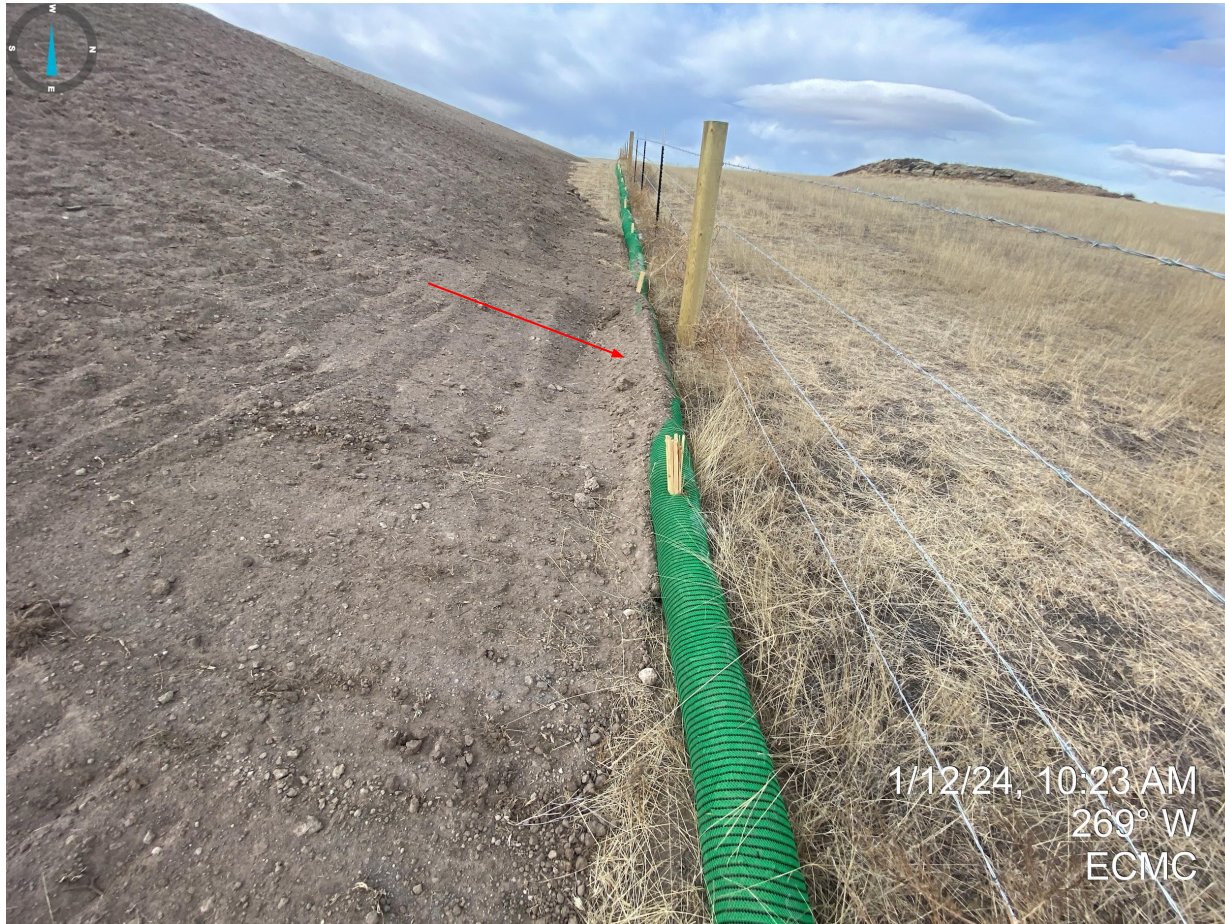
Photo 4. Northside of stockpile. Sediment controls (filtrexx) require maintenance.
