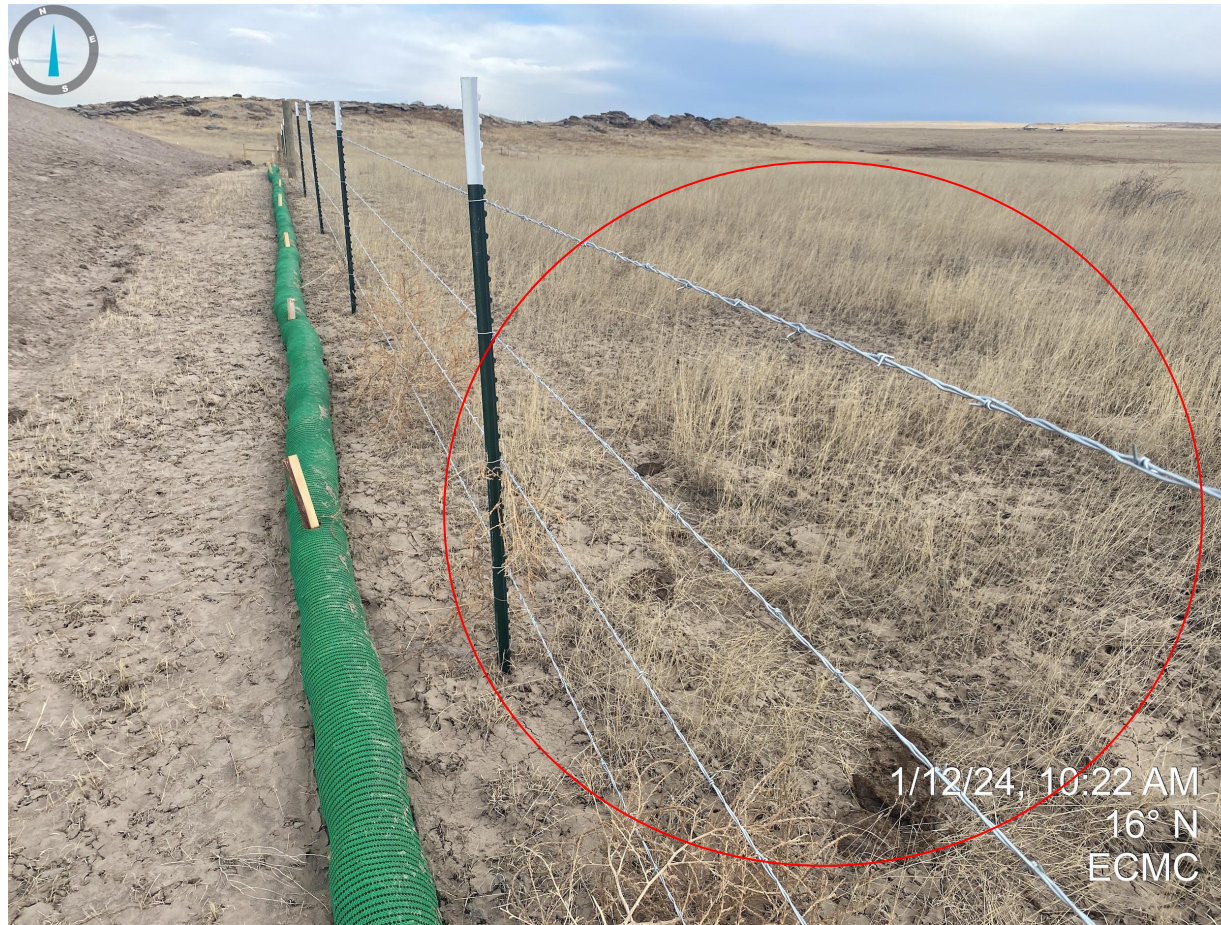
Photo 6. East side of stockpile. Evidence of wind erosion (soil deposition) outside of the fenced disturbance area resulting from unstabilized soils on the construction site.
