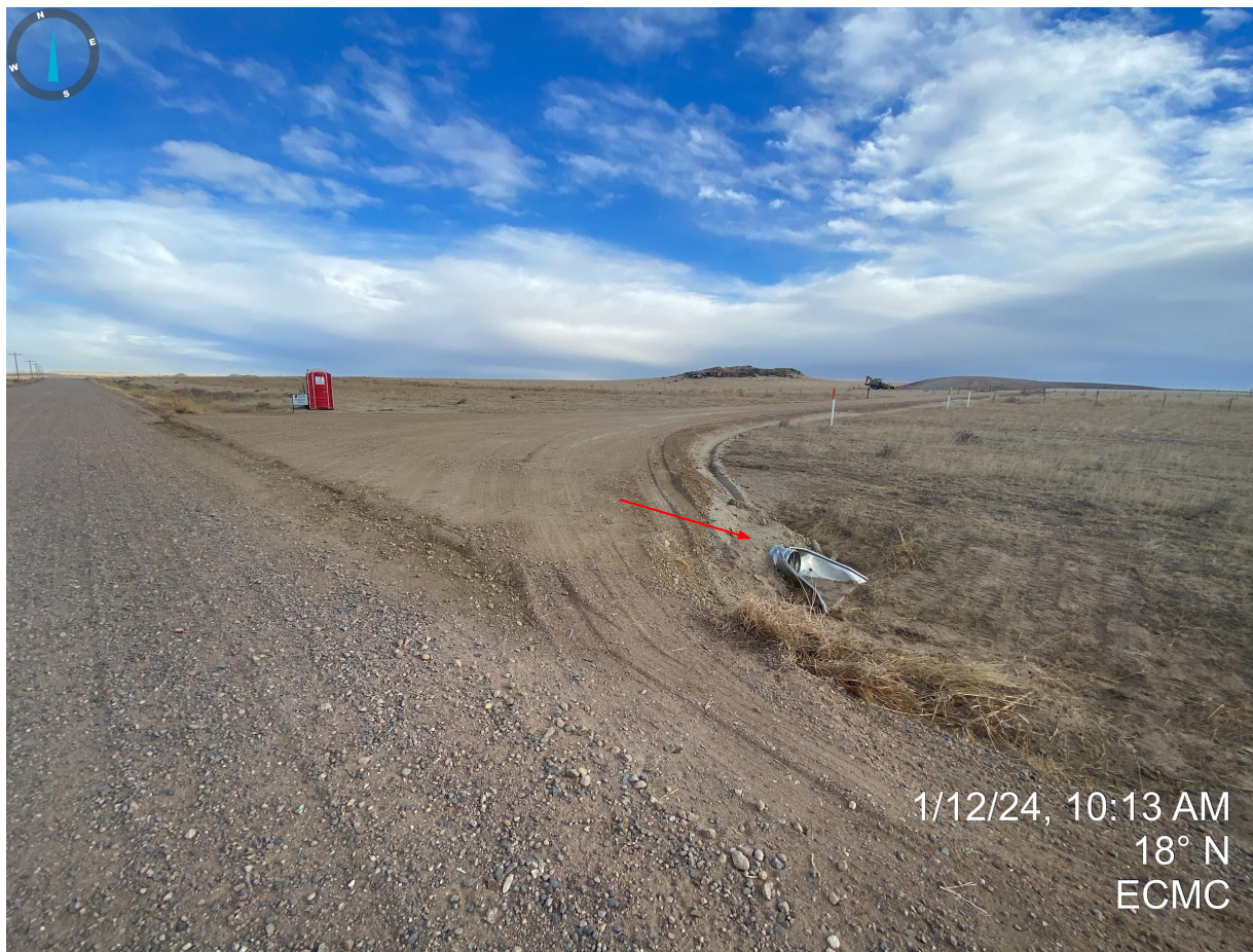
Photo 1. Soil around the culvert ends has been left unconsolidated; soils around the inlet/outlet don't appear to be compacted or otherwise stabilized.
