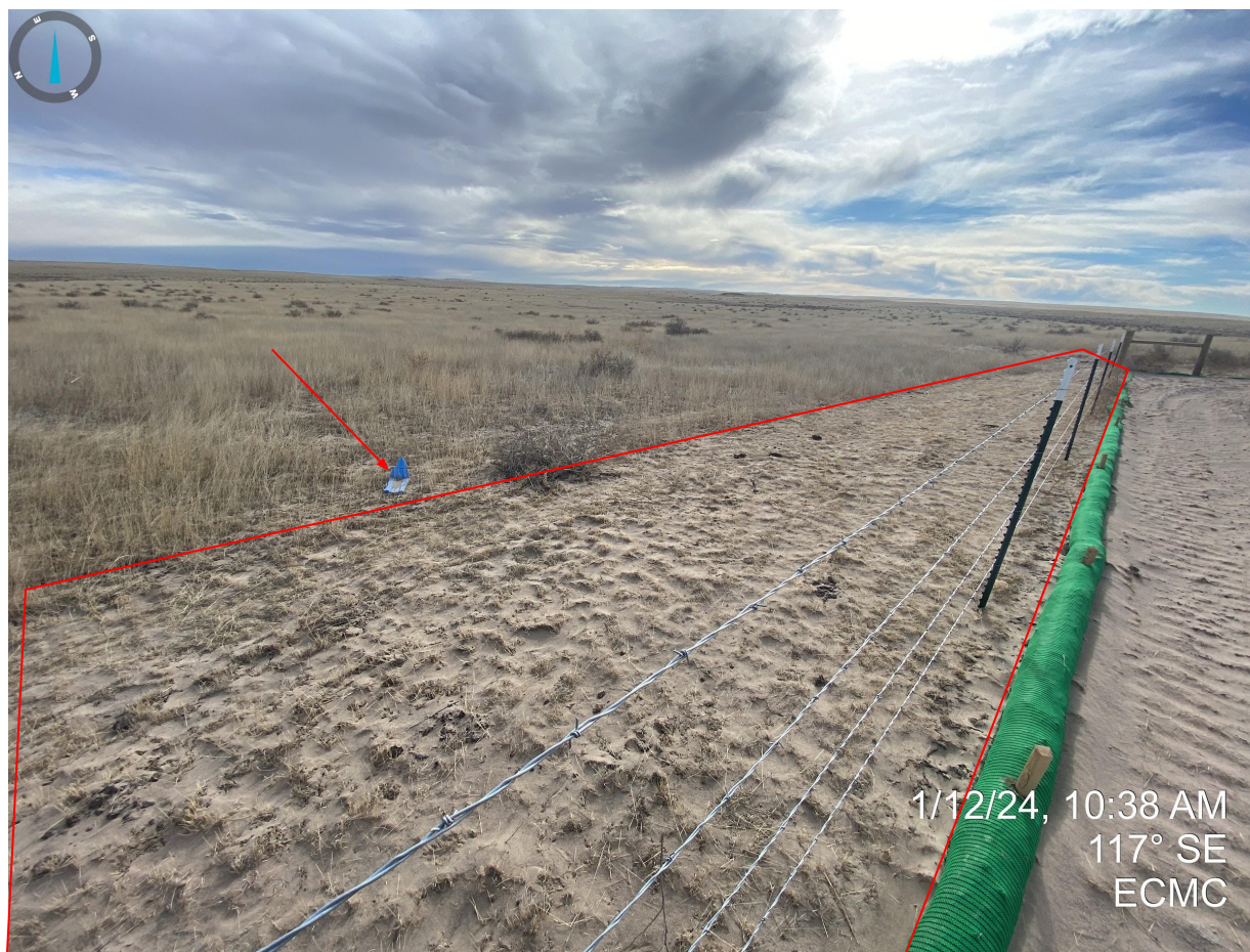
Photo 10. Continued from Photo 9. East side of pad construction. Evidence of wind erosion (soil deposition) outside of the fenced disturbance area resulting from unstabilized soils on the construction site. Also pictured (red arrow) trash/debris.
