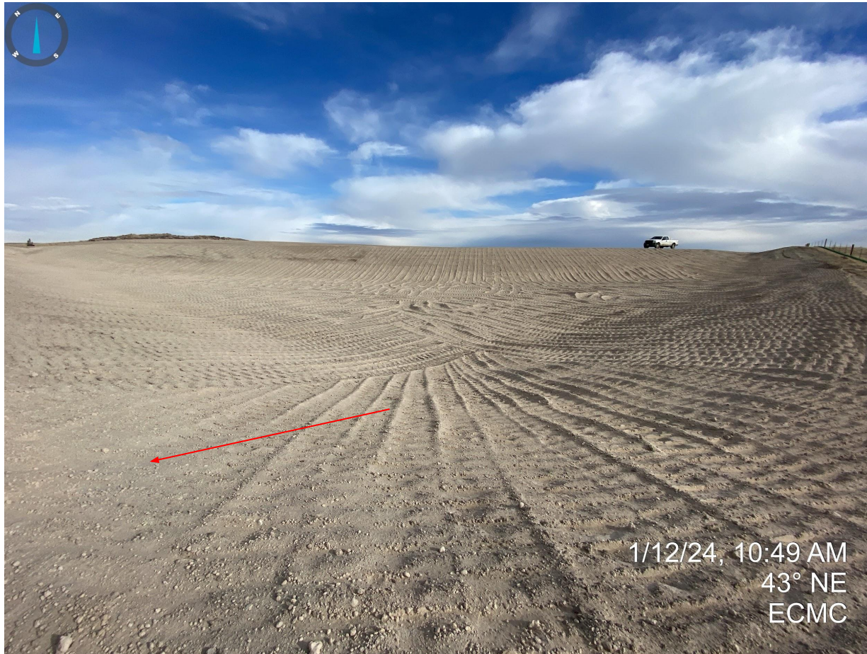
Photo 23. Southwest retention area. See comment in Photo 22. Red arrow indicates example of unstabilized soils.
