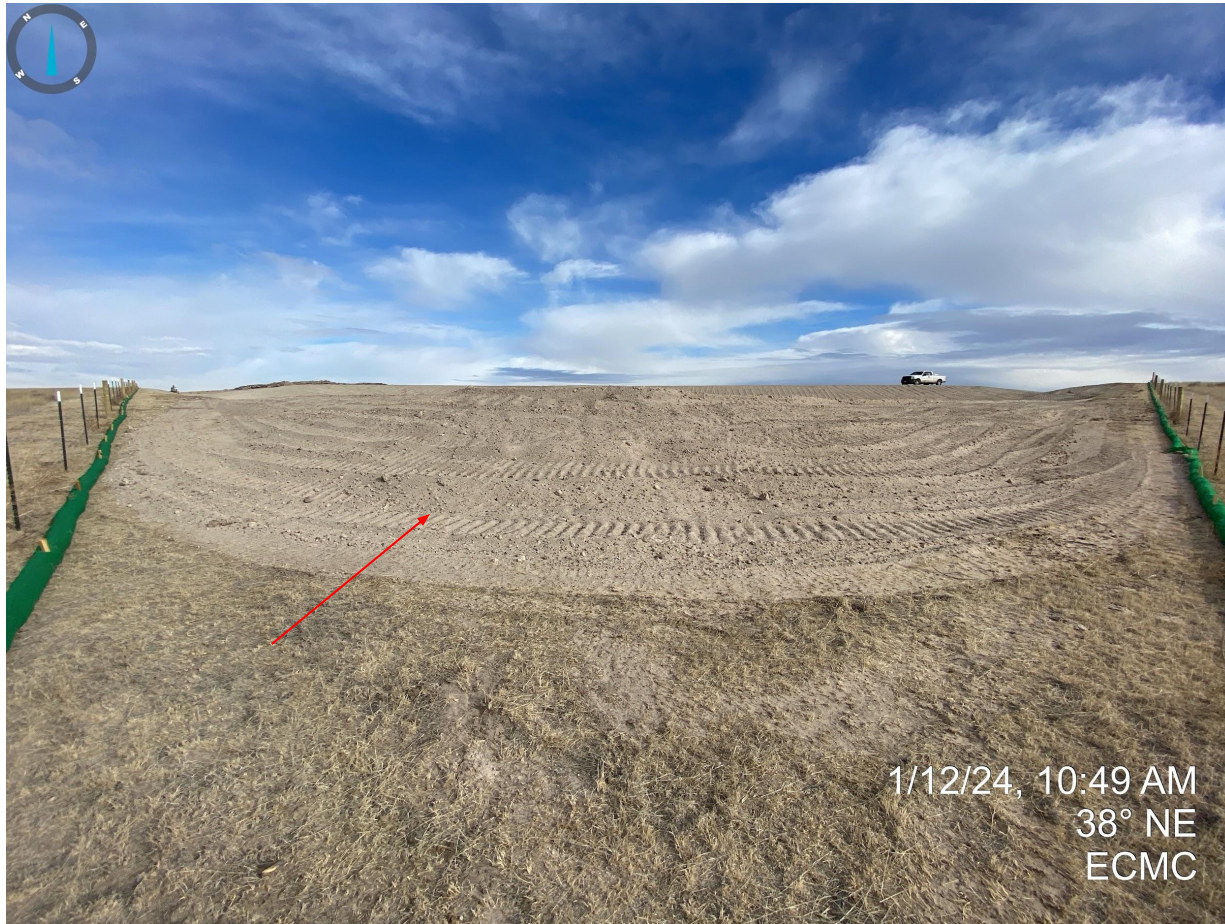
Photo 24. Improper equipment tracking (parallel to slope) on the backside of the stormwater retention area.
