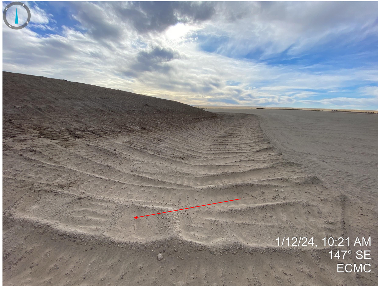
Photo 3. Northeast corner of drilling area, near stockpile. Stormwater ditches have been equipment tracked, however, tracks are beginning to fill with soil which indicates additional stabilization BMPs are required.
