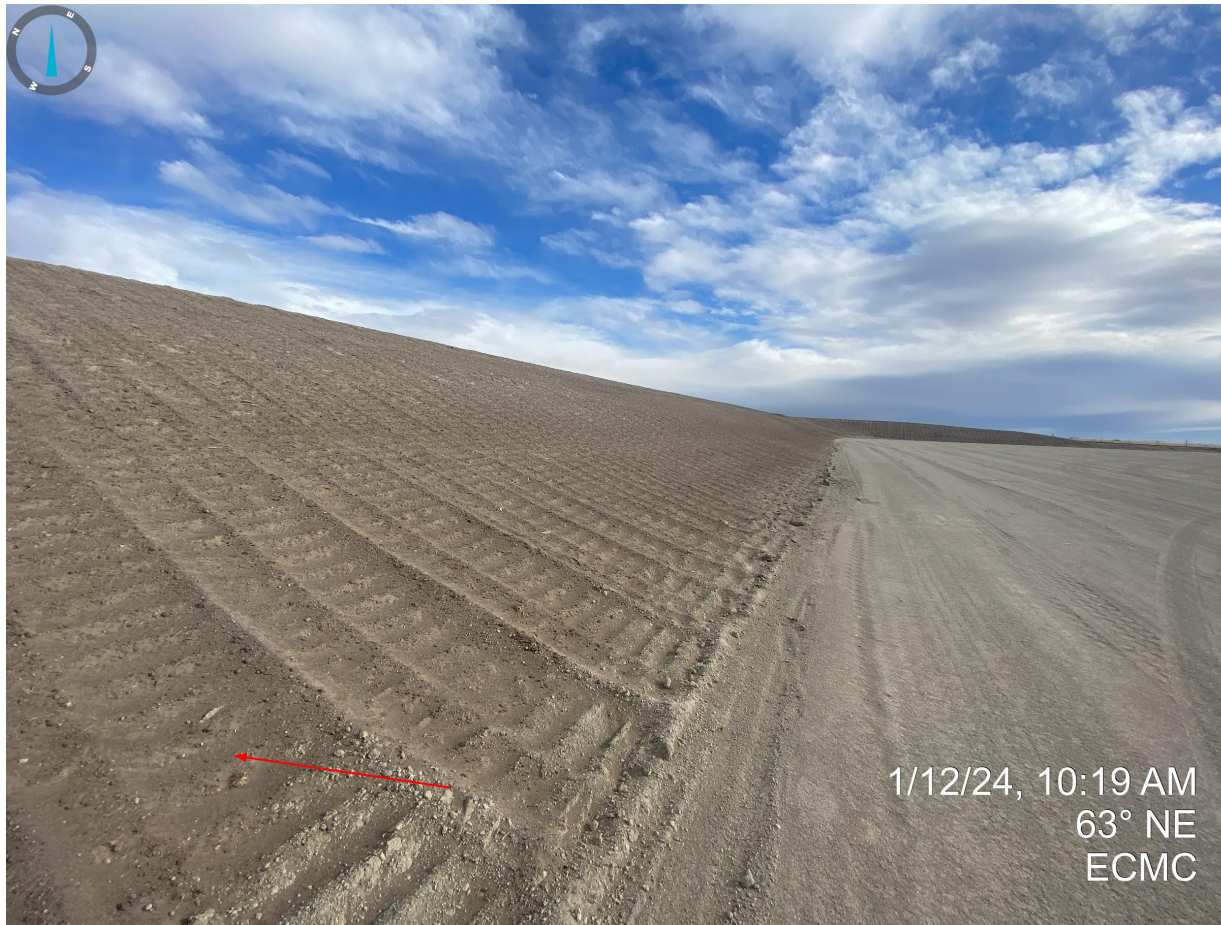
Photo 2. West side of topsoil stockpile. It appears the stockpile has been temporarily stabilized with evidence of equipment tracking, however, tracks are beginning to fill with soil which indicates additional stabilization BMPs are required.
