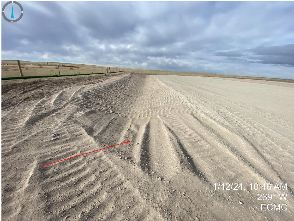
Photo 21. Unstabilized soils along the southern stormwater ditch.
