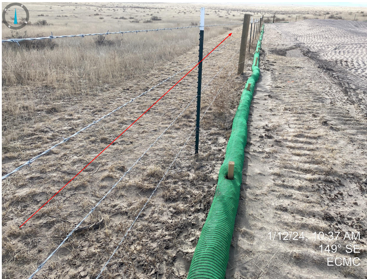
Photo 9. East side of pad construction. Evidence of wind erosion (soil deposition) outside of the fenced disturbance area resulting from unstabilized soils on the construction site.
