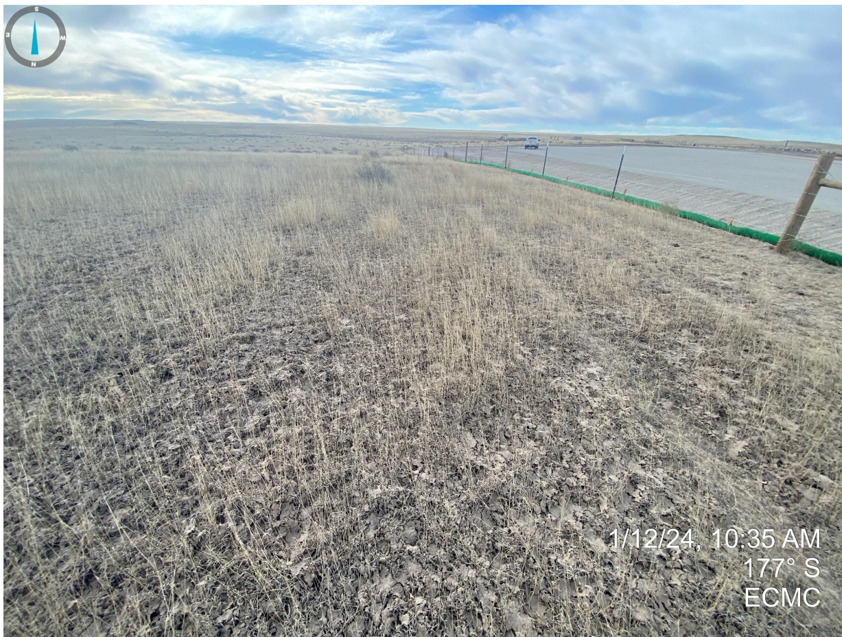
Photo 8. East side of pad construction, outside of the disturbance area. Evidence of wind erosion (soil deposition) outside of the fenced disturbance area resulting from unstabilized soils on the construction site.
