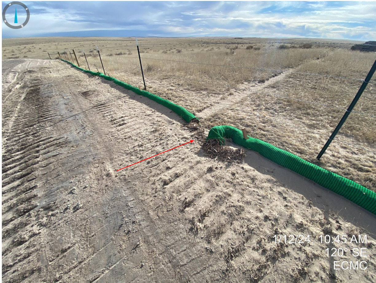
Photo 17. Southeast corner of location. Filtrexx requires repair/replacement.
