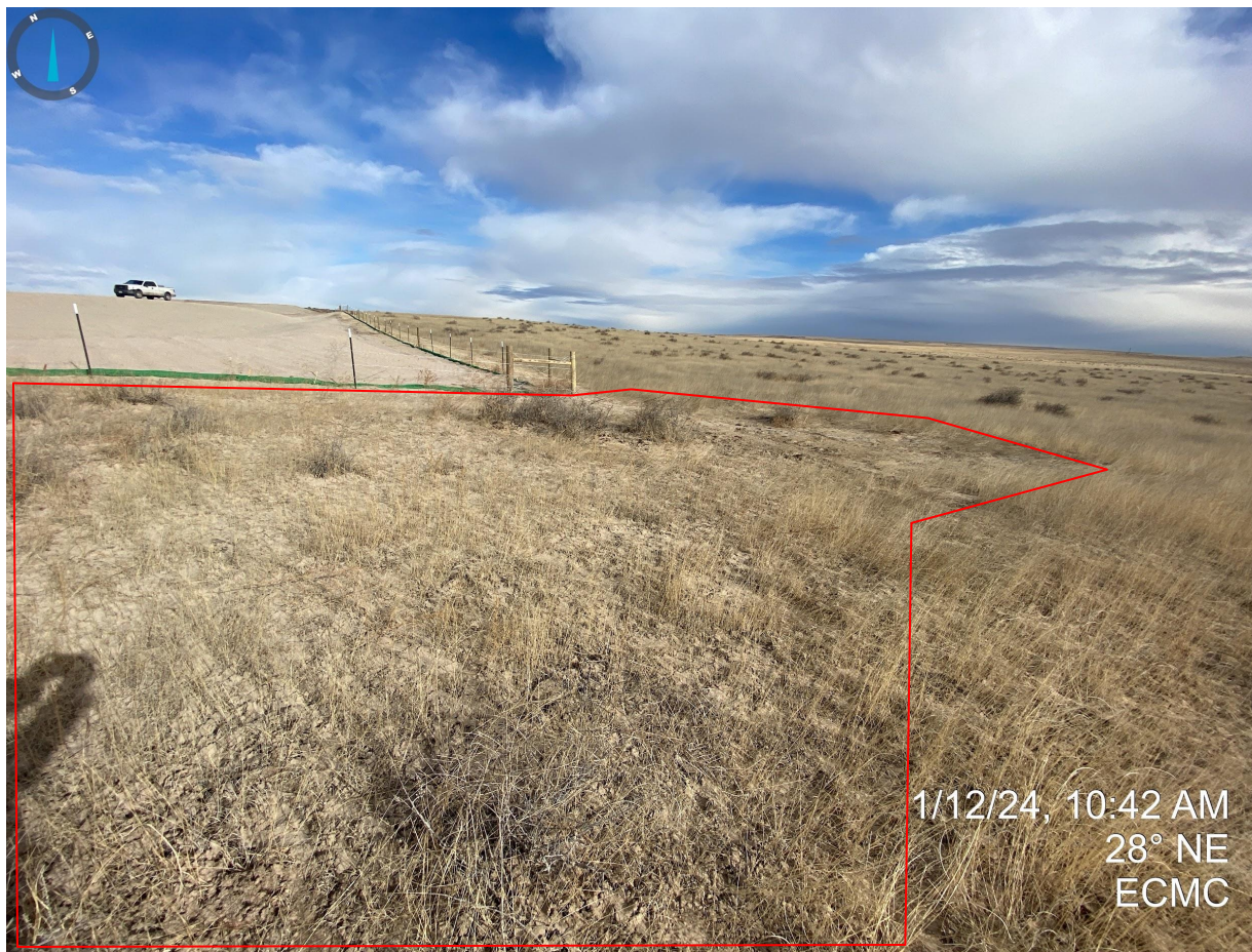
Photo 14. Southeast side of pad construction, outside of fenced disturbance area. Evidence of wind erosion (soil deposition) outside of the fenced disturbance area resulting from unstabilized soils on the construction site. Red polygon is only an approximation of new disturbance.
