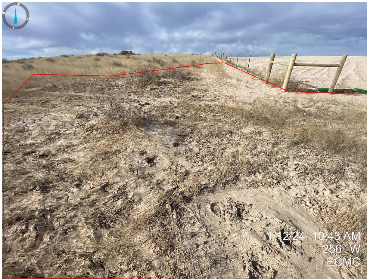
Photo 13. Southeast side of pad construction, outside of fenced disturbance area. Evidence of wind erosion (soil deposition) outside of the fenced disturbance area resulting from unstabilized soils on the construction site. Red polygon is only an approximation of new disturbance.
