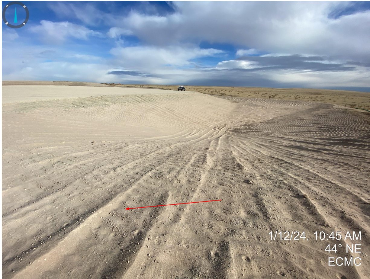
Photo 20. Southeast retention area. See comment in Photos 18 & 19. Red arrow indicates example of unstabilized soils.
