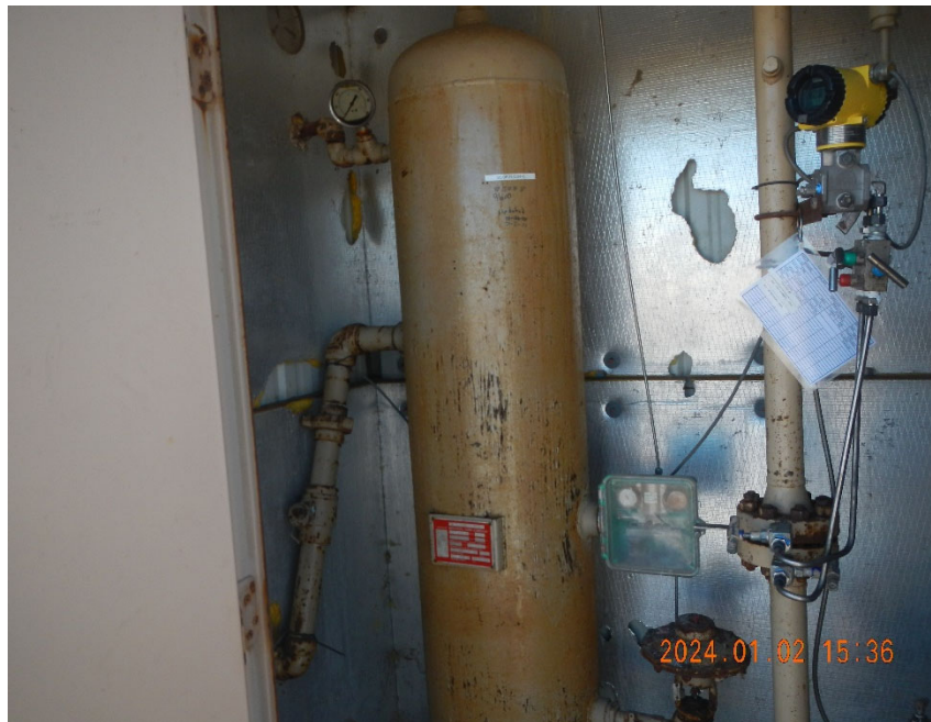
5. Vertical separator inside meter shed.
