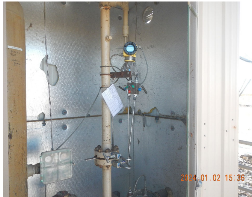
6. Digital gas meter inside meter shed.
