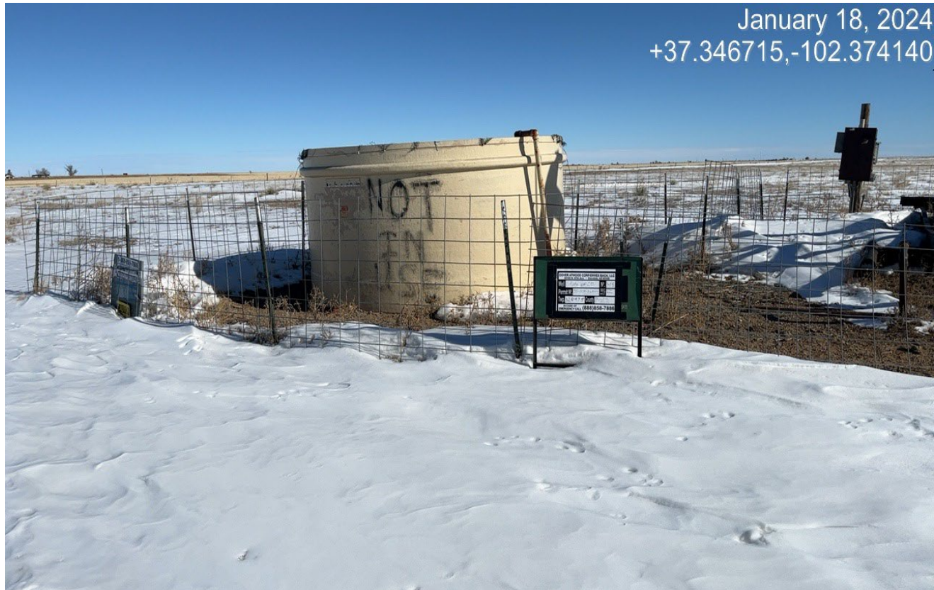
Photo 2. Facing toward the open top tank. There is not secondary containment at the tank and there is oily fluids inside the tank.
