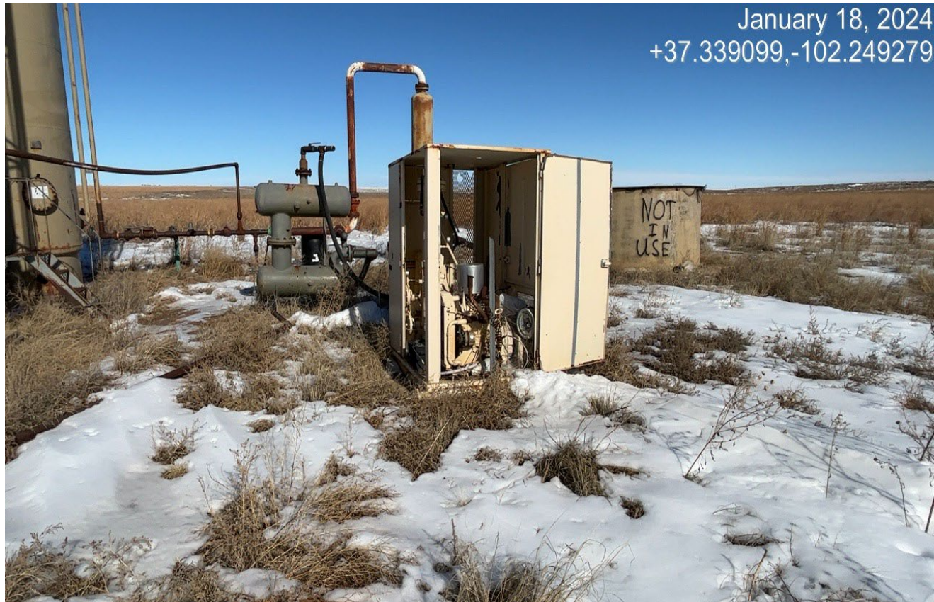
Photo 7. There is equipment not maintained and weeds grown around the equipment. Door has fallen off this shed. Previous corrective action is not completed.
