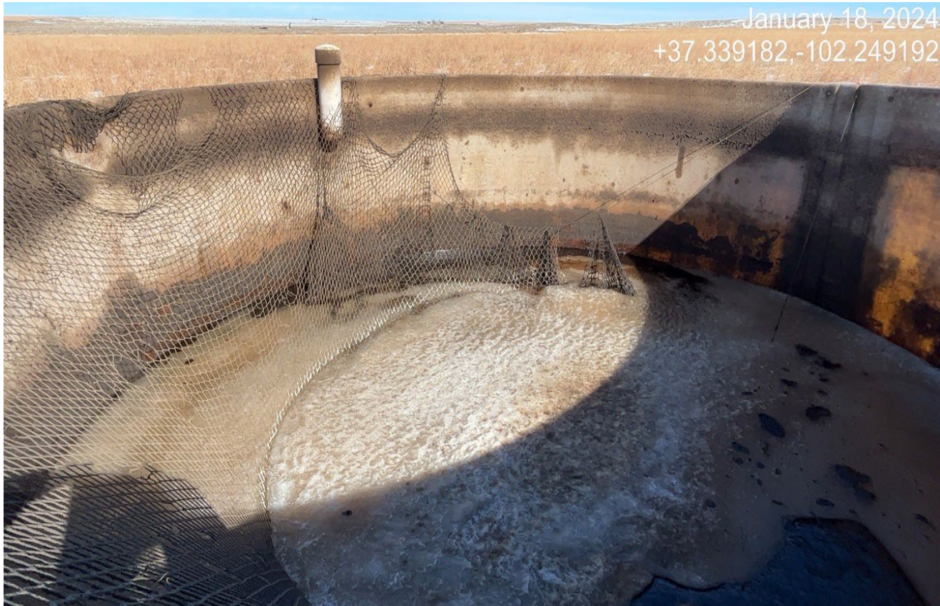
Photo 9. There is liquid in the tank and the netting is in disrepair.
