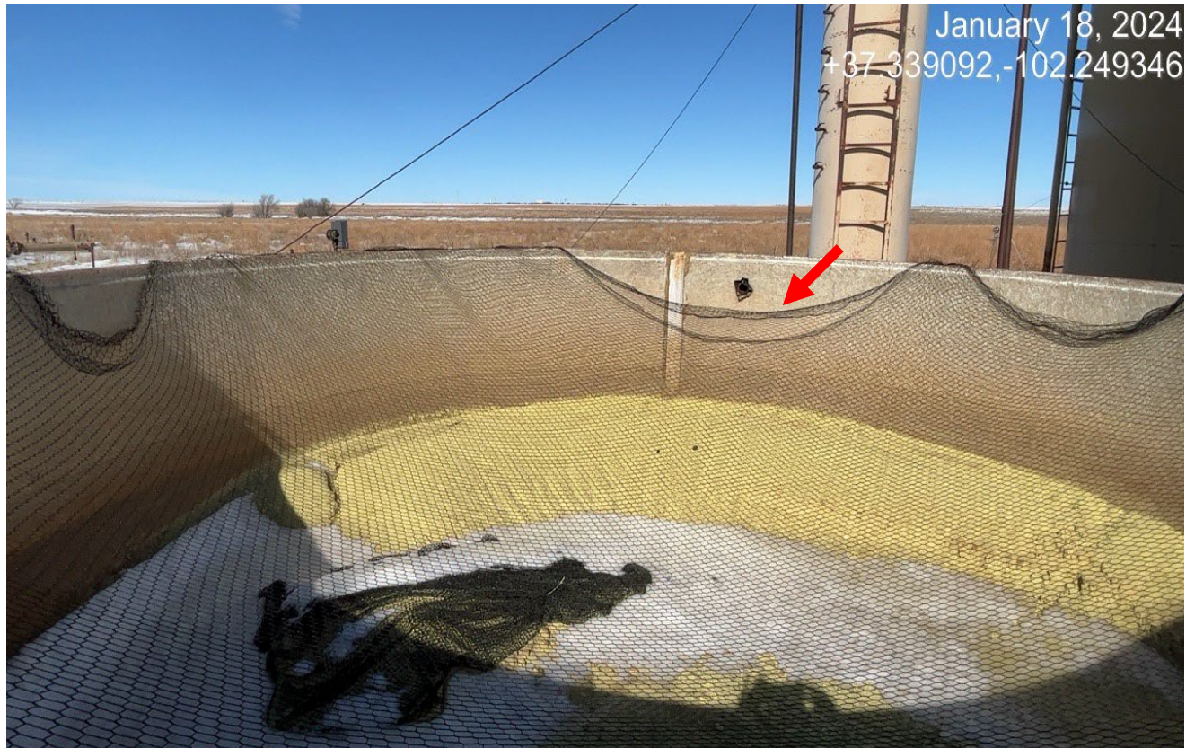
Photo 5. The netting on the open top tank has come uncovered on the edges which wildlife could gain entry.
