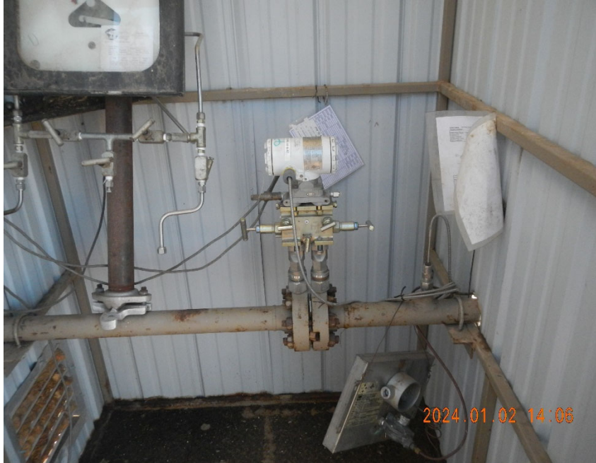
5. Digital gas meter inside meter shed.
