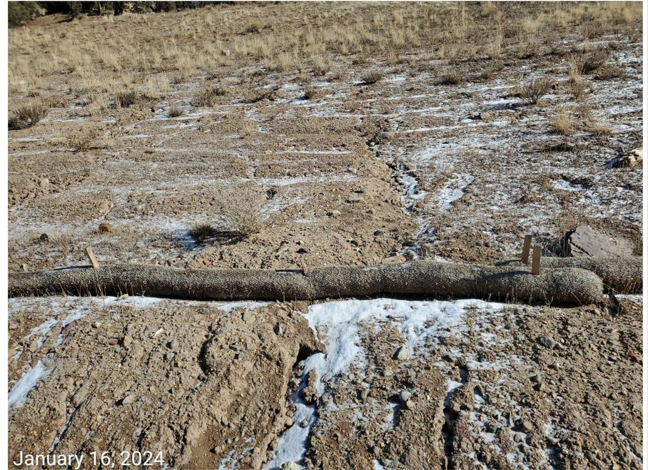
**Photo 4:** Photos taken from the eastern working pad surface of the well site. Photos examples of interim areas not progressing towards 1003 standards. Photos also examples showing stormwater and erosion control BMPs are missing or insufficient; BMPs to minimize erosion and degradation within the interim areas are inadequate; erosion log (wattles) has not been installed or maintained per good engineering practices resulting stormwater cutting beneath the BMP and degradation to the ditch.
