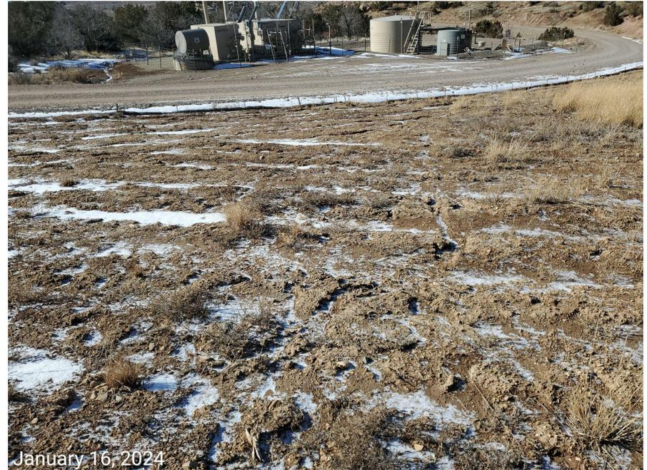
**Photo 8:** Photos taken from the western interim areas of the well site. Photos examples of interim areas not progressing towards 1003 standards. Photos also examples showing stormwater and erosion control BMPs are missing or insufficient; BMPs to minimize erosion and degradation within the interim areas are inadequate. Additional reclamation effort and stormwater management required in these areas.
