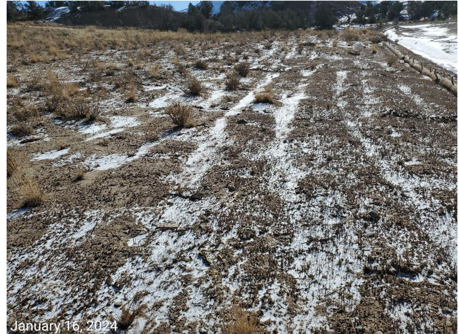
**Photo 5:** Photos taken from the eastern interim areas of the Location. Photos examples of interim areas not progressing towards 1003 standards. Photos also examples showing stormwater and erosion control BMPs are missing or insufficient; BMPs to minimize erosion and degradation within the interim areas are inadequate. Additional reclamation effort and stormwater management required in these areas.
