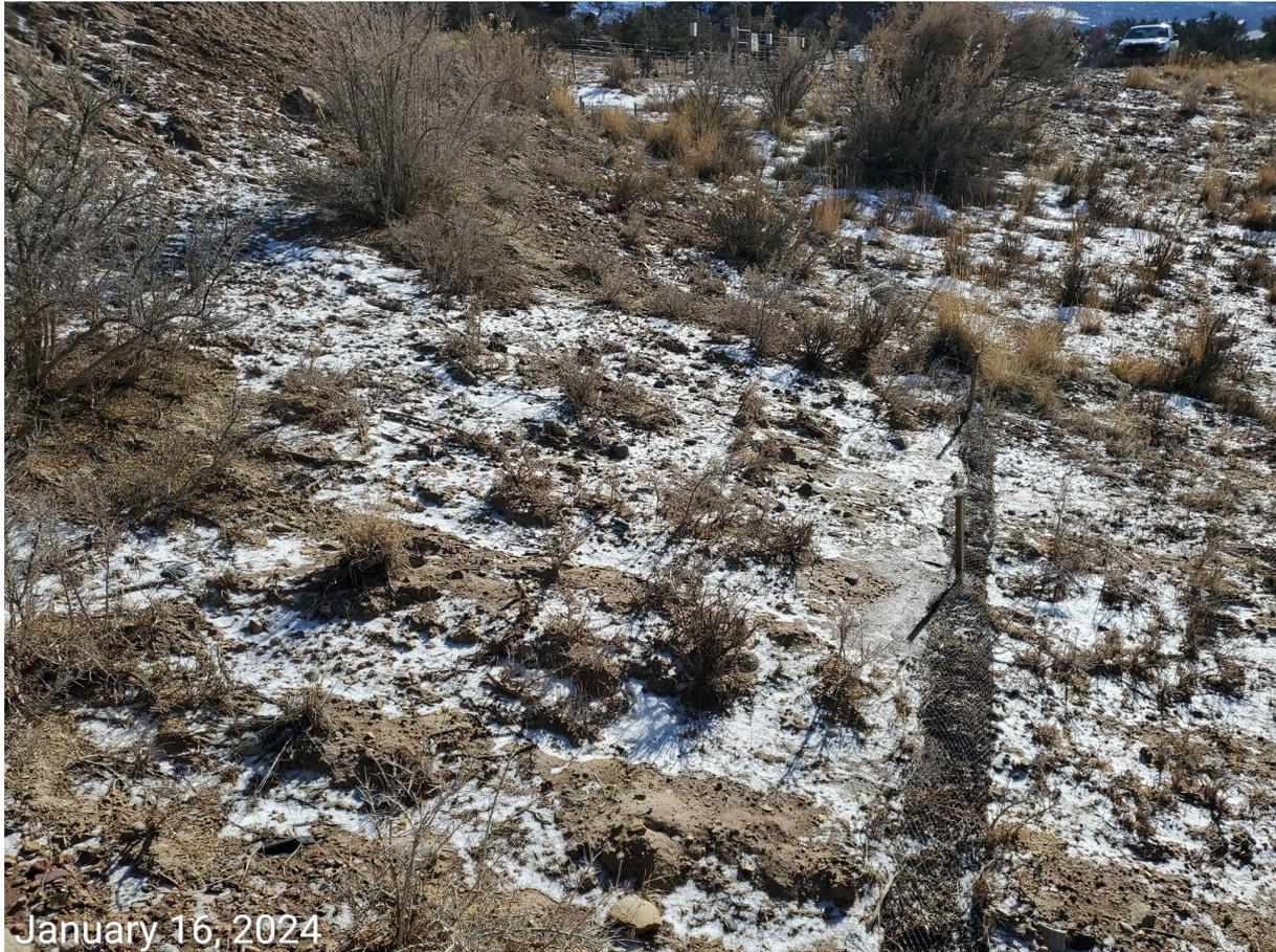
**Photo 7:** Photo example of erosion logs that have not been maintained in proper functioning condition. Erosion logs implemented appear to also be made of plastic material; this is an improper control, considered trash/debris and requires removal.
