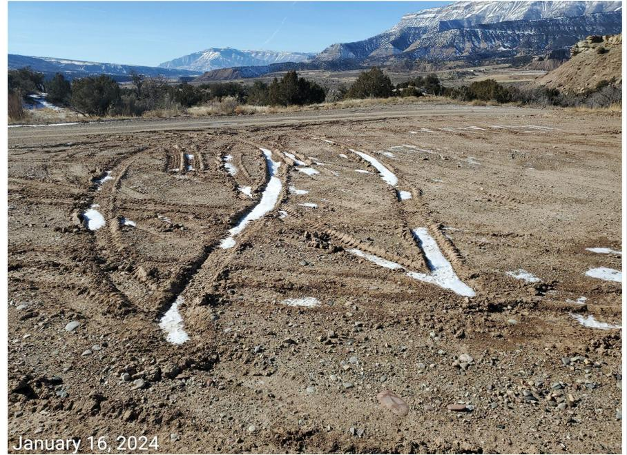
**Photo 3:** Photos examples showing BMPs to stabilize the working pad surface, as well as to minimize erosion, degradation and off-site sediment transport are missing or insufficient.
