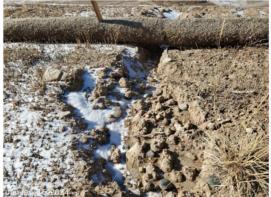
**Photo 6:** Erosion logs have not been installed or maintained in accordance with good engineering practices; stormwater has cut under the BMP resulting in concentrated flows and erosion degradation.
