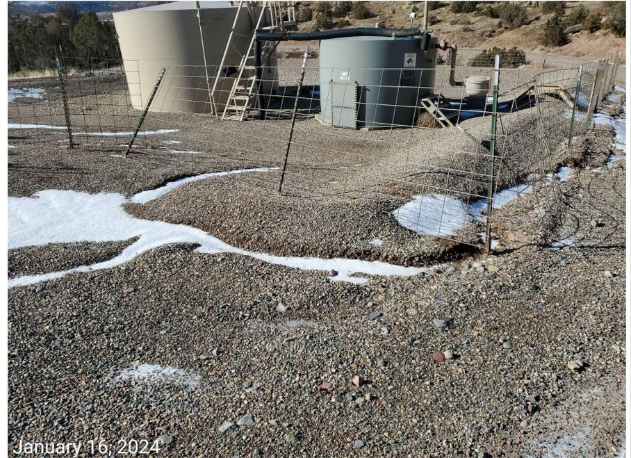
**Photo 9:** Photo taken from the tank battery facility. Photo shows erosion degradation due to stormwater runoff. Photo also shows fence at battery in disrepair.
