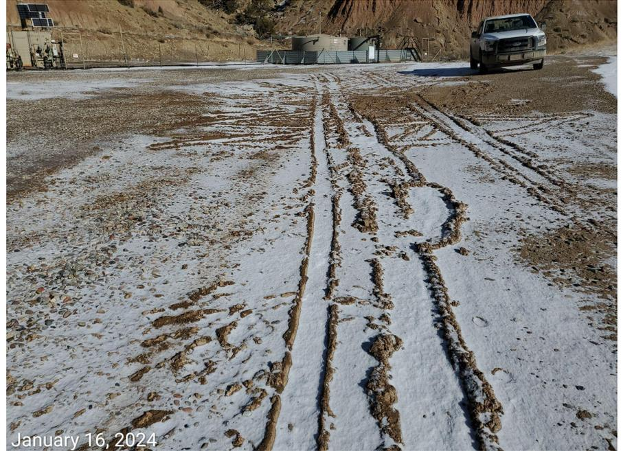
**Photo 3:** Photos taken examples showing BMPs to stabilize the working pad surface, as well as to minimize erosion, degradation and off-site sediment transport are missing or insufficient.
