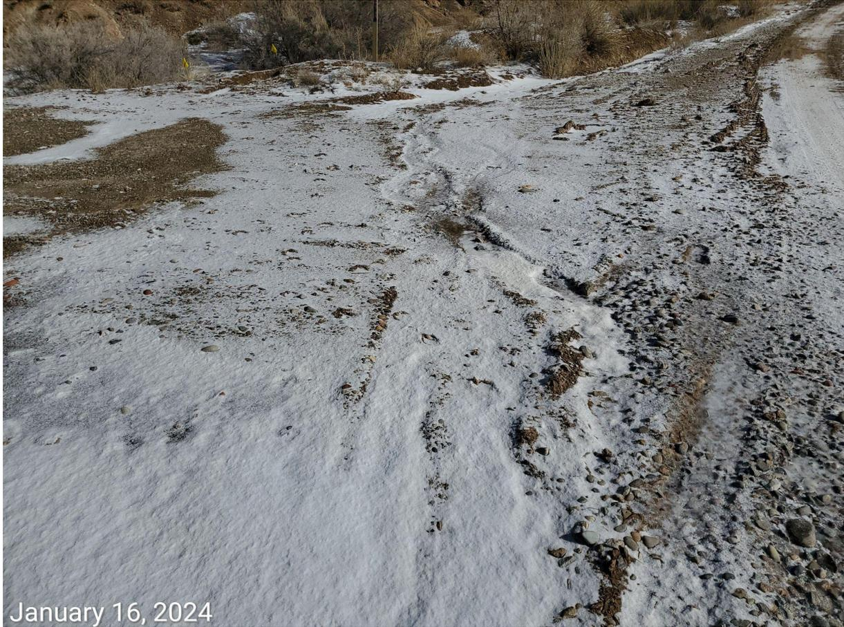
**Photo 5:** Photo taken from the north end of the Location; stormwater runoff from the working pad surface is resulting in erosion and degradation.
