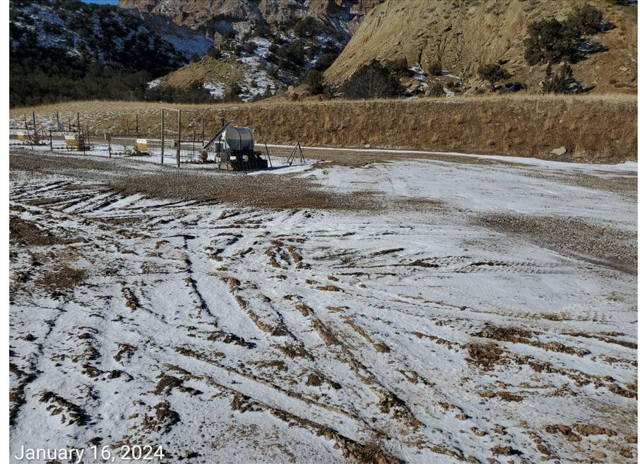
**Photo 1:** Photos 1-2 taken from the southern working pad surface of the Location. Photos provide an overview of the Location from southwest, west, north to northeast. Photos also examples showing BMPs to stabilize the working pad surface, as well as to minimize erosion, degradation and off-site sediment transport are missing or insufficient.
