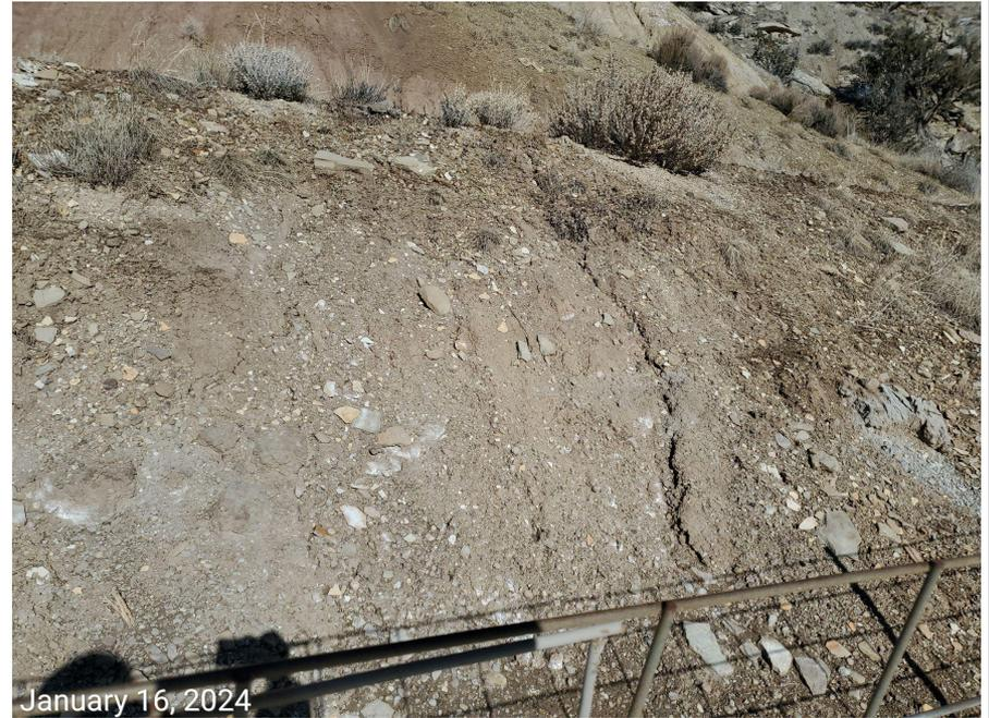
**Photo 4:** Photos taken from the slopes behind the tank battery facility. Stormwater and erosion control BMPs are missing or insufficient. Soil are bare and erosion degradation is apparent. Sediment eroded from the slopes are deposited within a ditch, which discharges off-site.
