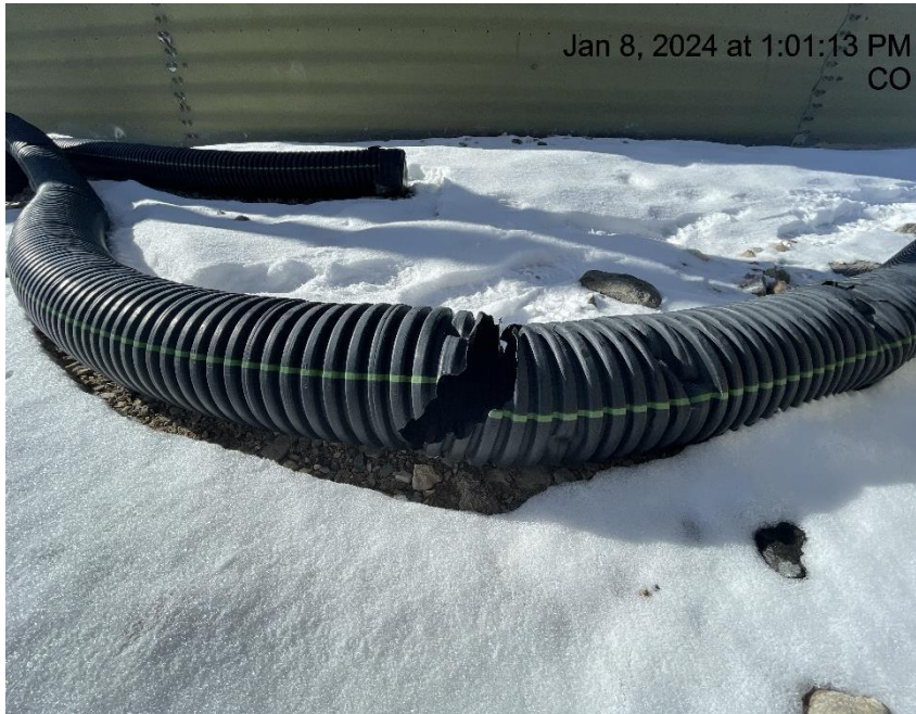
Photo # 2038 From inspection 708902741 hole in flowline heating insulation/wildlife hazard
