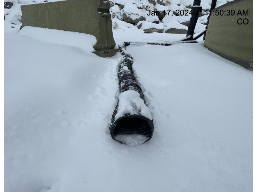
Photo # 2975 Flowline heating insulation open ended
