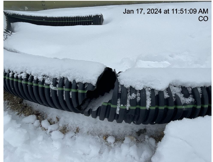
Photo # 2976 Hole in flowline heating insulation/wildlife hazard
