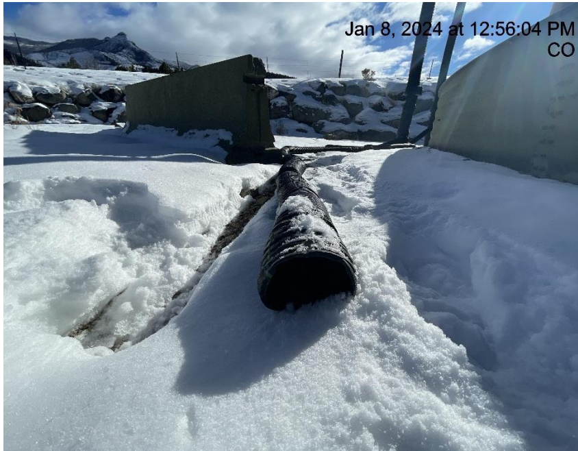
Photo # 2037 From inspection 708902741 flowline heating insulation open ended
