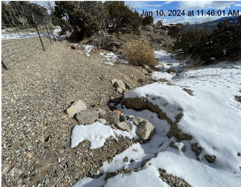
Photo # 2270 Check dams needs maintenance
