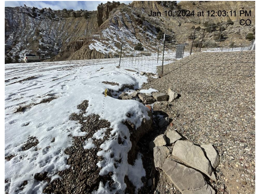
Photo # 2273 Check dam needs maintenance
