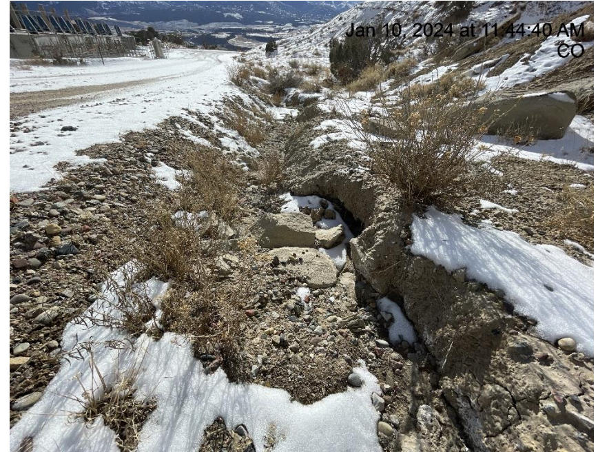
Photo # 2269 Check dam needs maintenance
