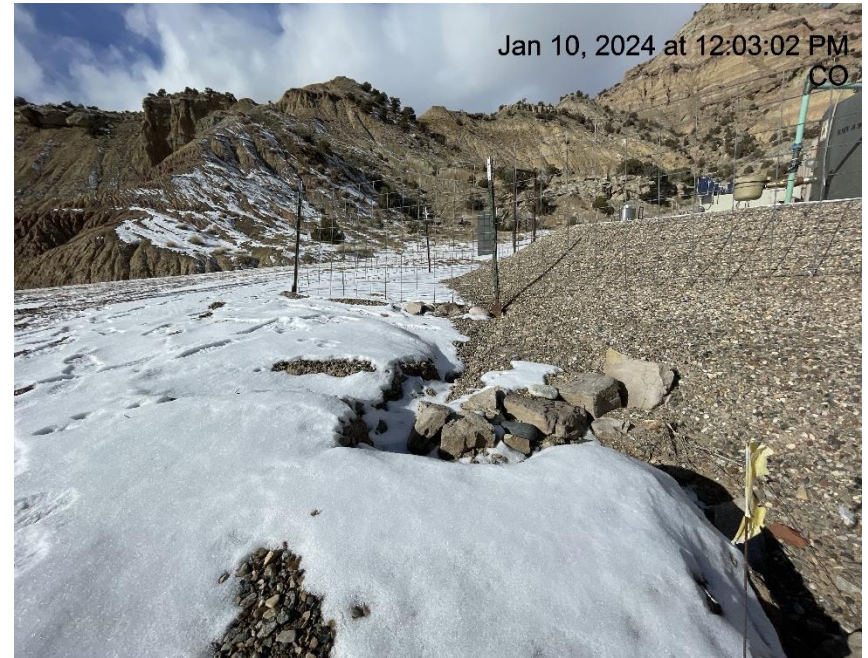
Photo # 2271 Check dam needs maintenance
